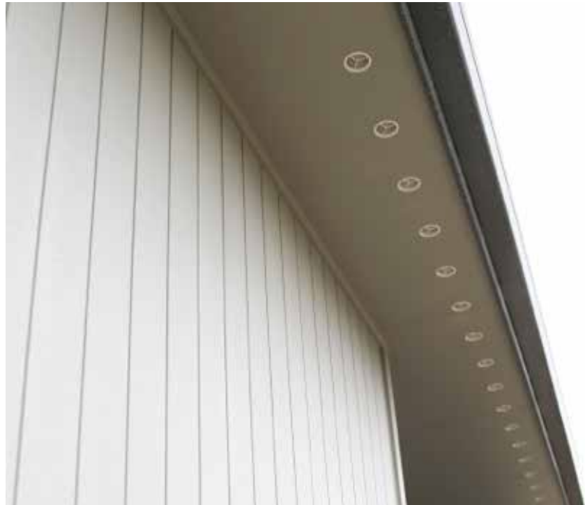
Skillion roof with ventilation openings under the eaves
