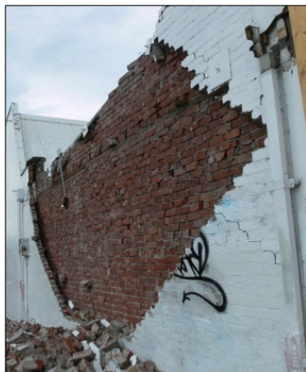
(c) Typical two-way bending collapse of outer layer
