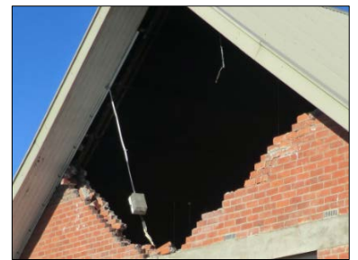
(c) Gable end walls – partial collapse (perimeter top restraint)
