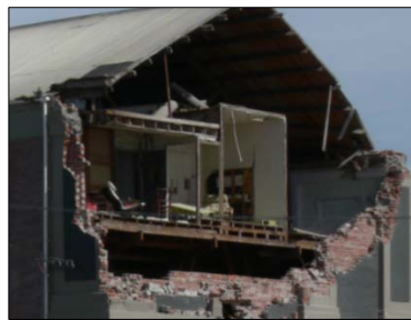
(b) Gable end walls - full collapse cantilever failure (no top restraint)
