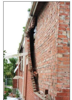
(e) Side view of wall displacement - 2
