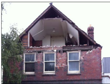
(a) Gable end walls – cantilever failure (no top restraint)
