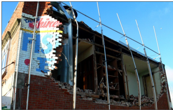
(h) Two-way bending collapse of wall having two single leafs- 2
