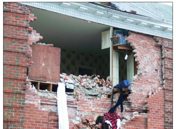
(b) Collapse in two-way bending of a cavity wall of two single leafs
