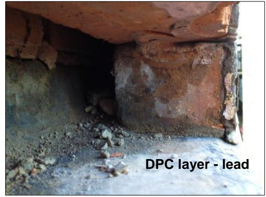
(c) Exterior cavity wall with brick removed, exposing the lead damp-proof course and air gap cavity
