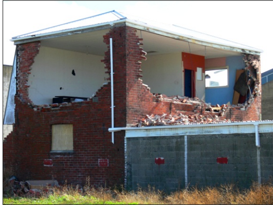
(f) Example of combined failure modes
