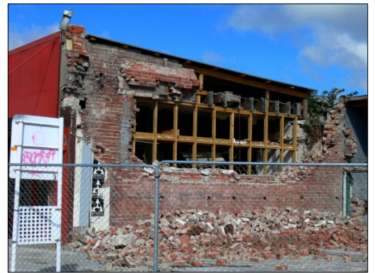
(i) Two-way bending collapse of wall having two single leafs - 3
