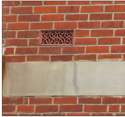
(b) Typical cavity wall air vents
