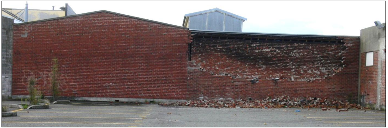
Figure 27 – Comparison of two cavity walls. Weak lime mortar with badly corrode cavity ties and poor top restraint (right), cement mortar and adequate top support, cavity tie condition unknown (left)
