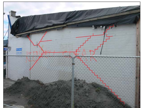
(b) Two-way typical cracking pattern (highlighted in red for clarity)
