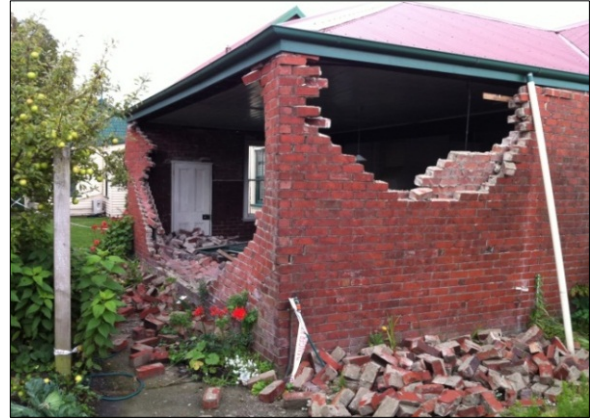
(g) Collapse in two-way bending of a wall with two single leafs - 1
