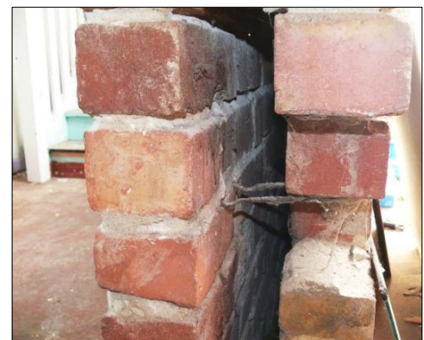
(b) Typical cavity wall cross-section showing metal ties
