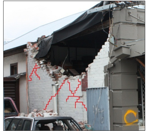
(b) Short spanning cavity walls with unrestrained top boundary support (highlighted in red for clarity)
