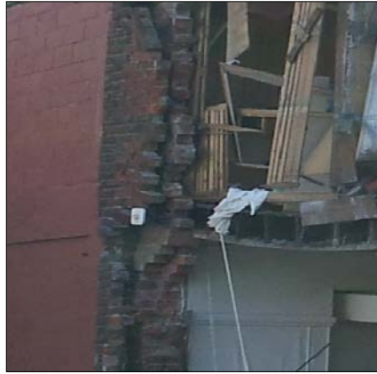
(a) Continuous outer and inner wall layer
