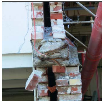
(a) RC beam extending across both inner and outer wall layer
