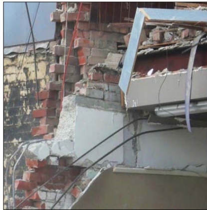
(a) RC beam on inner wall layer
