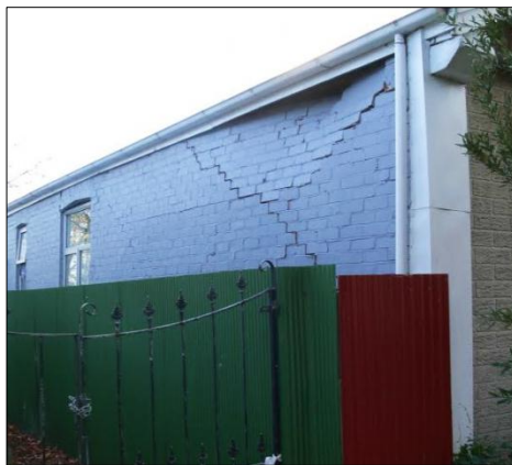
(a) Typical two-way cracking pattern - onset of collapse of top portion
