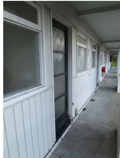
Figure 22. Cable runs (in plastic conduits) from base of central unit door to adjacent units.
