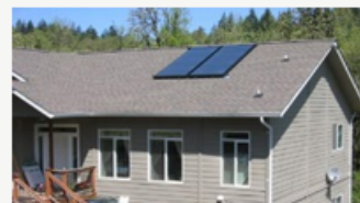
Solar hot water (using flat plate)
