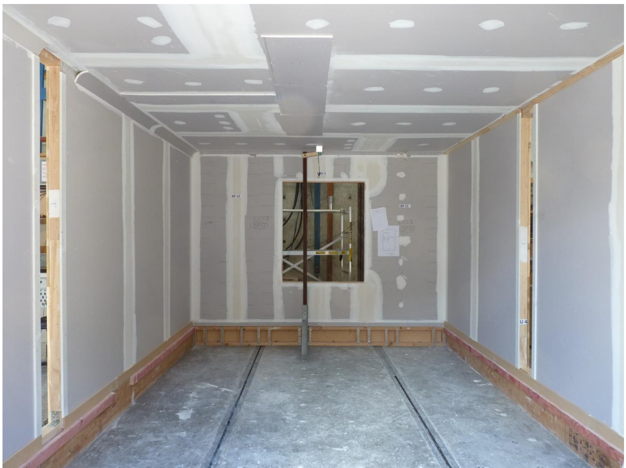
Figure 3. Internal view of test room before testing commenced
