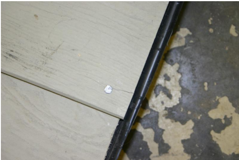
Figure A.15 Cracking of Weatherboards
