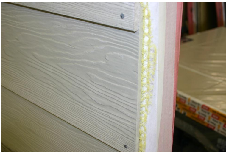
Figure A.8 Face Nailing of Weatherboards
