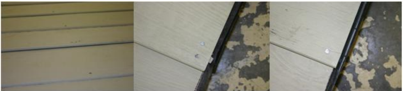
Figure 17 Bulging, Nailthrough and Cracking of Claddings
