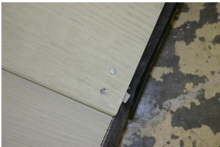
Figure A.16 Nailthrough Required a Second Nail to be Used Here
