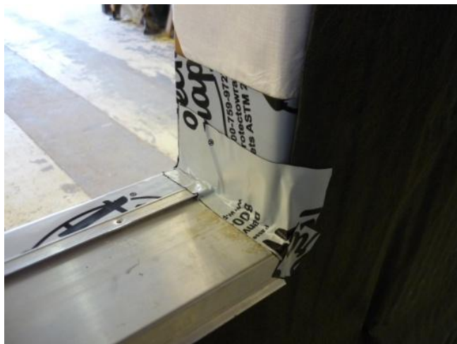
Figure 9 Window Sill Tray Details for Drainage Planes
