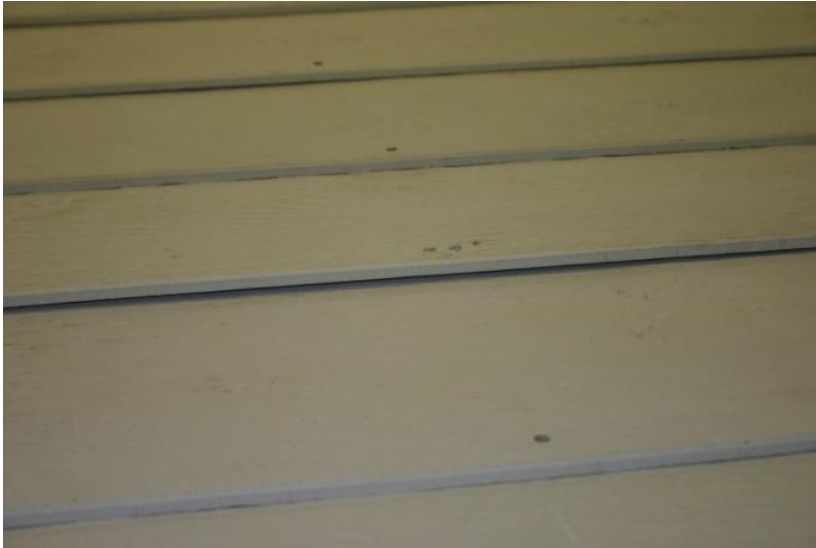
Figure A.14 Bulge in Weatherboards
