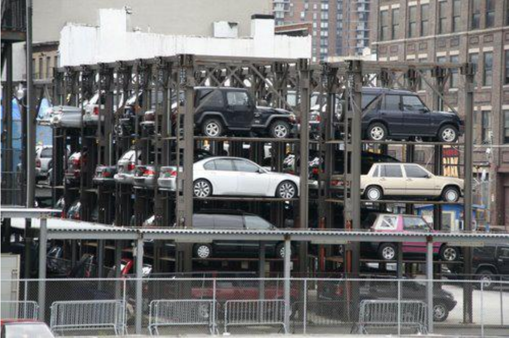
Figure 44: Outdoor stacking four-vehicles high in New York City
