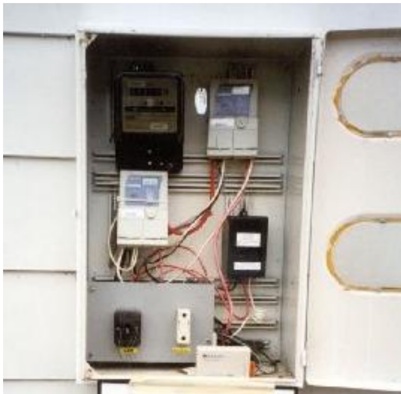
Figure 7. The hot water and total household electrical energy use being monitored by Siemens S2AS meters
