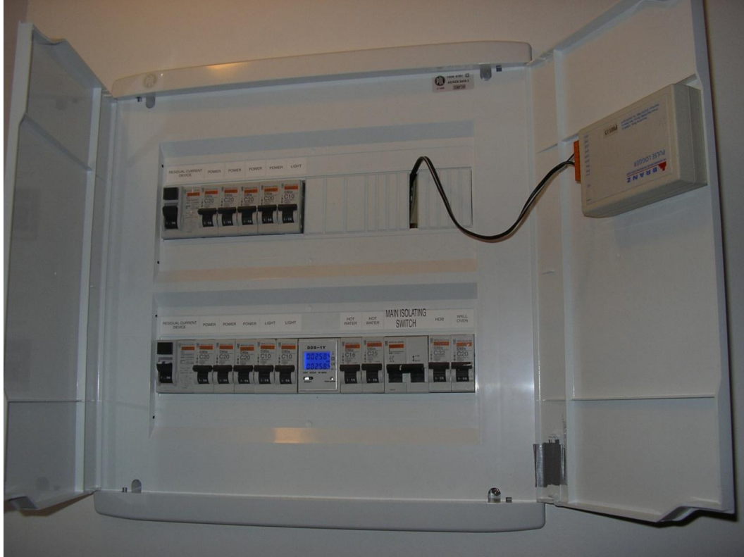
Figure 8. A DDS1Y DIN rail electricity meter (blue display) measuring a heat pump water heater installed on a typical modern fuse-board
