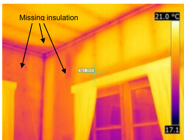
Figure 17: Area of insulated ceiling included in the image as a reference for the wall insulation
