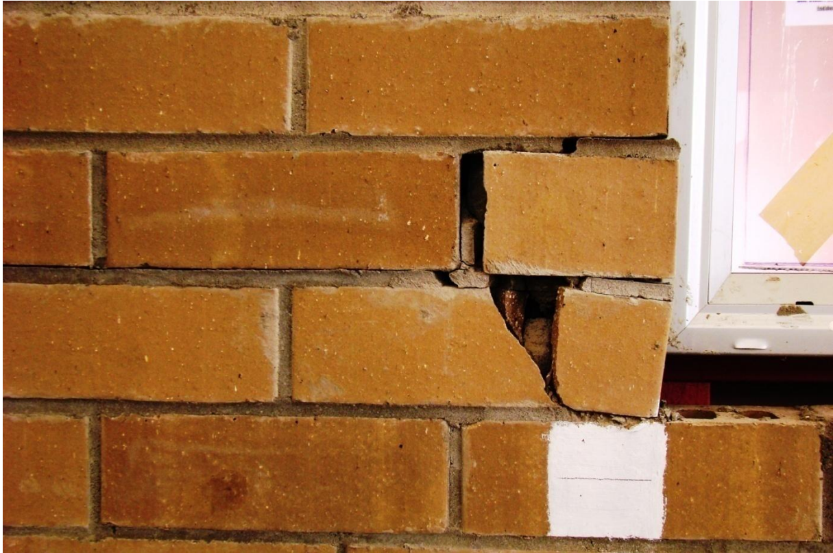
Figure 95. Brick damage in Side 1 lower-storey veneer at Window S1A in Stage G
