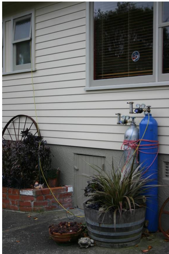
Figure 19. Picture of the tracer gas cylinders located outside the building for safety reasons.
