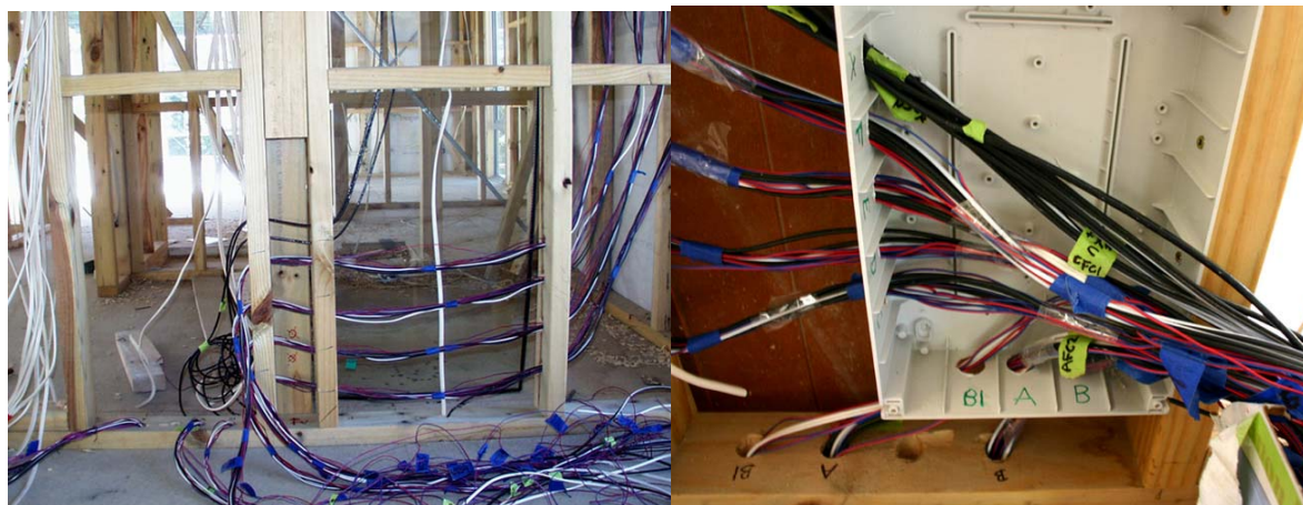
Figure 11. Where the monitoring wires come together – logging cupboard during construction.
