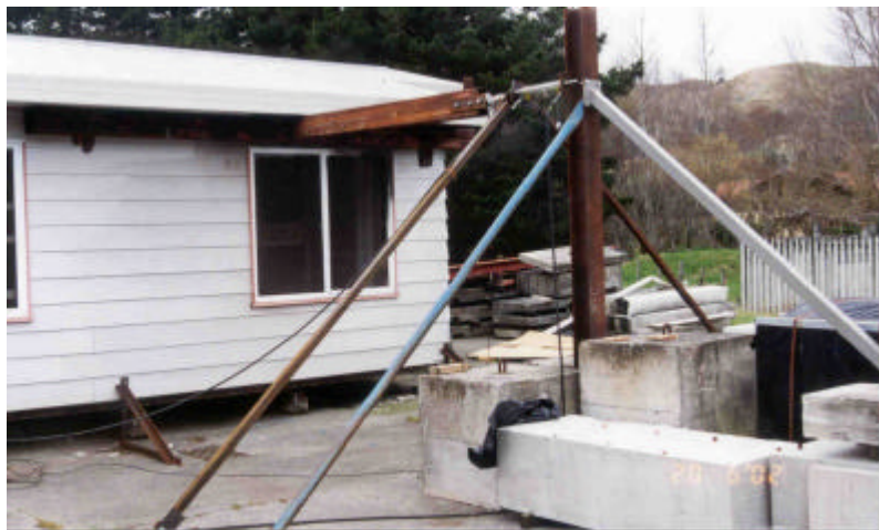
(g) Loading rig on west end of house
