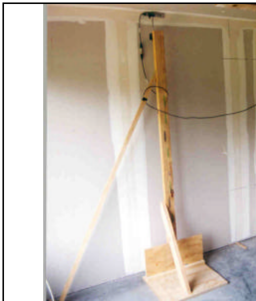
(e) Measurement of deflection of walls
