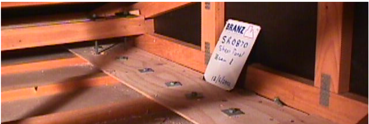
(c) Plywood strip in roof space to connect timber loading beams to wall top plate
