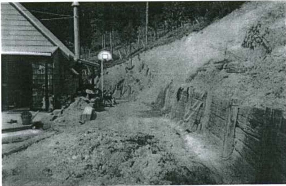
Figure D1: View showing slip debris against house
