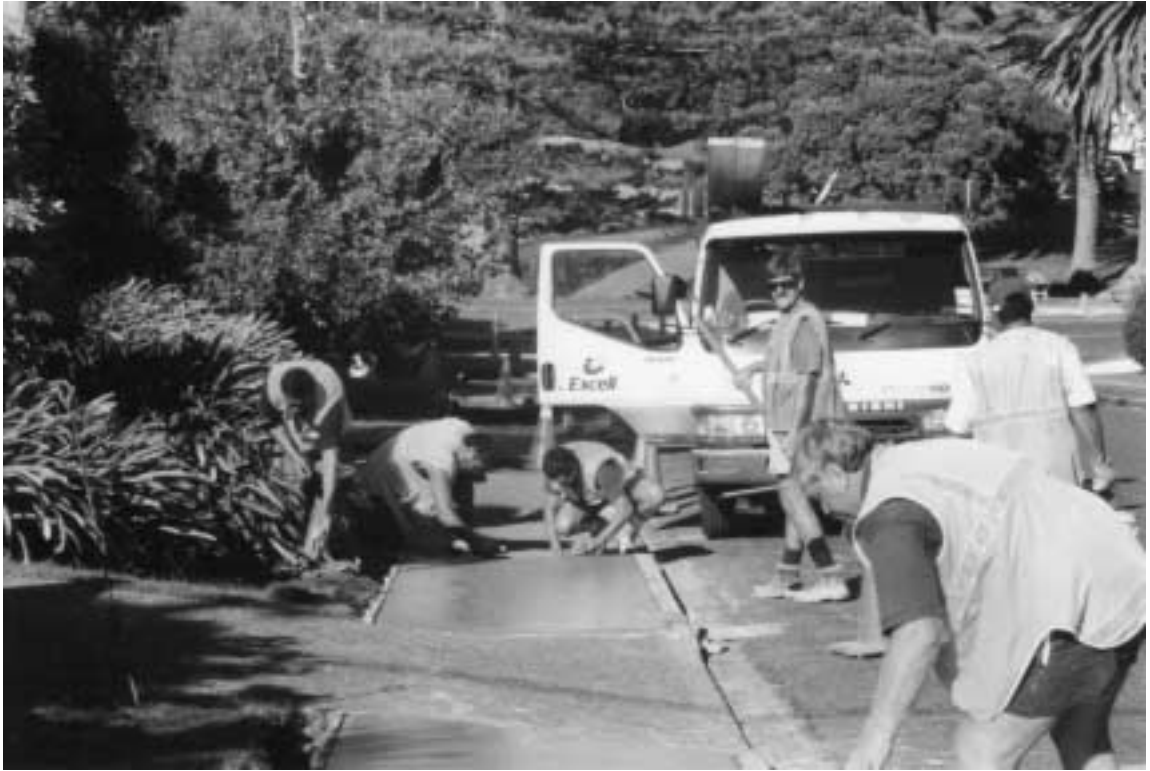
Figure 9 Finishing Recycled Aggregate Concrete Field Trial
