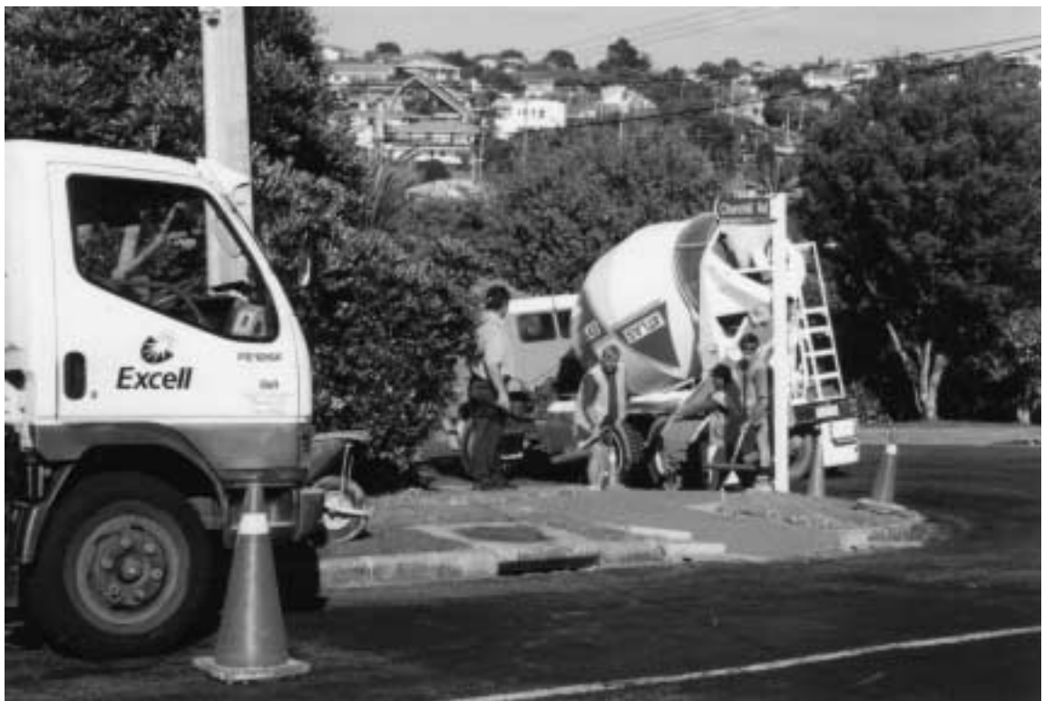
Figure 8 Placing Recycled Aggregate Concrete For Field Trial
