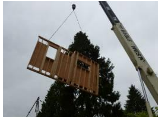
Figure 37: An open wall panel being craned into place in Vancouver, Canada (IDEAbuilder, 2014).
