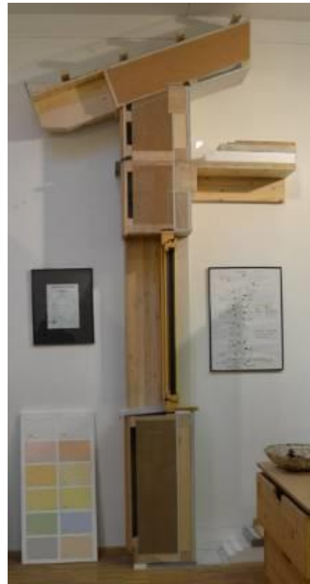
Figure 35: The walls of German and Austrian houses tend to be far thicker than New Zealand's and contain far more insulation.
