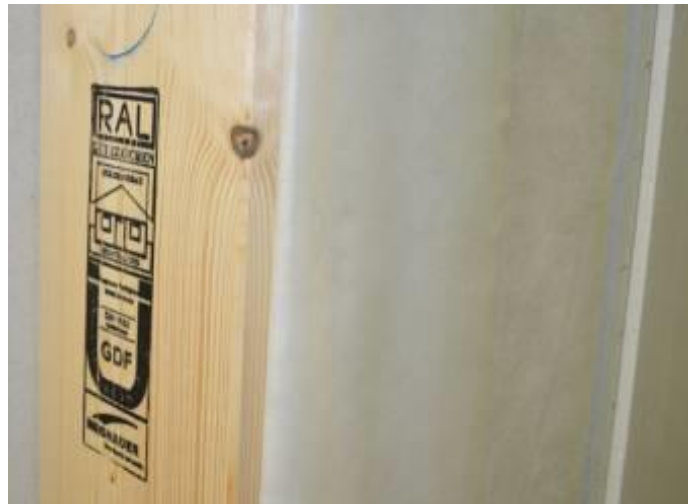
Figure 43: The RAL certification shows the building materials meet the minimum German standards.
