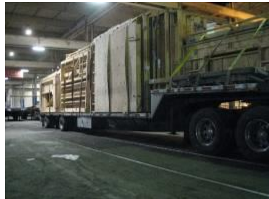
Figure 41: An open panel house ready for transport to site in Vancouver (IDEAbuilder, 2014).
