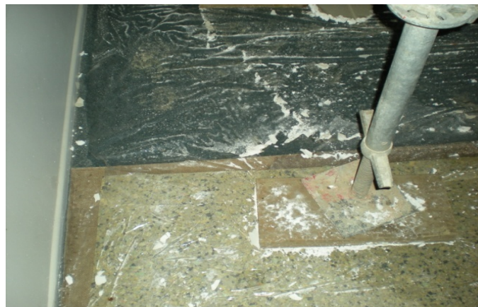
Figure 20: (Photo 15) Plastic wrapped carpets. Some owners opt to retain original carpets after remediation to cut down on repair costs.
