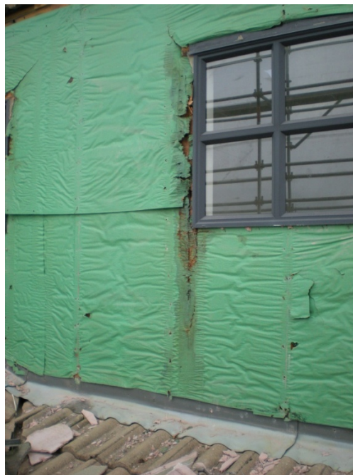
Figure 14: (Photo 5) Once cladding is removed water damage is often seen with the disintegration of building paper
