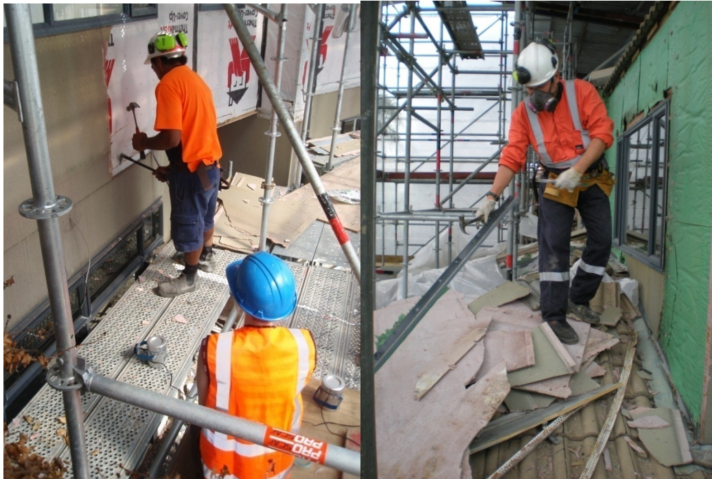
Figure 13: (Photo 3 & 4) The decladding process in Complex 1 – boards of cladding are pulled from the buildings by the remediators. This is thought to be a time of possible high spore exposure. Sampling machines can be seen in the foreground.
