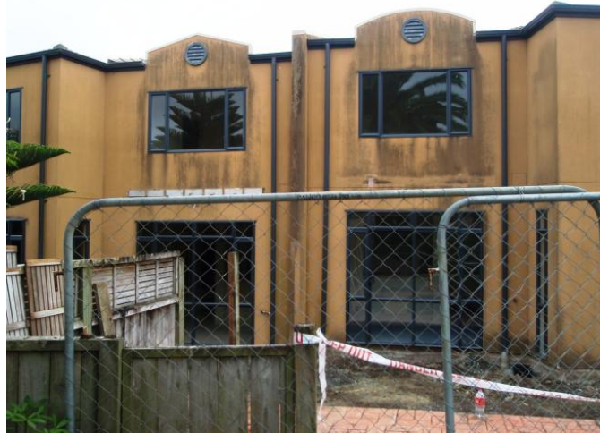
Figure 11: (Photo 1) Units in Complex 1 prior to remediation and scaffolding – dark areas of water damage are clearly visible as dark areas on the monolithic cladding
