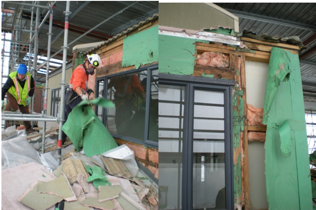
Figure 15: (Photo 6 & 7) Building paper and insulation layers are also removed.
