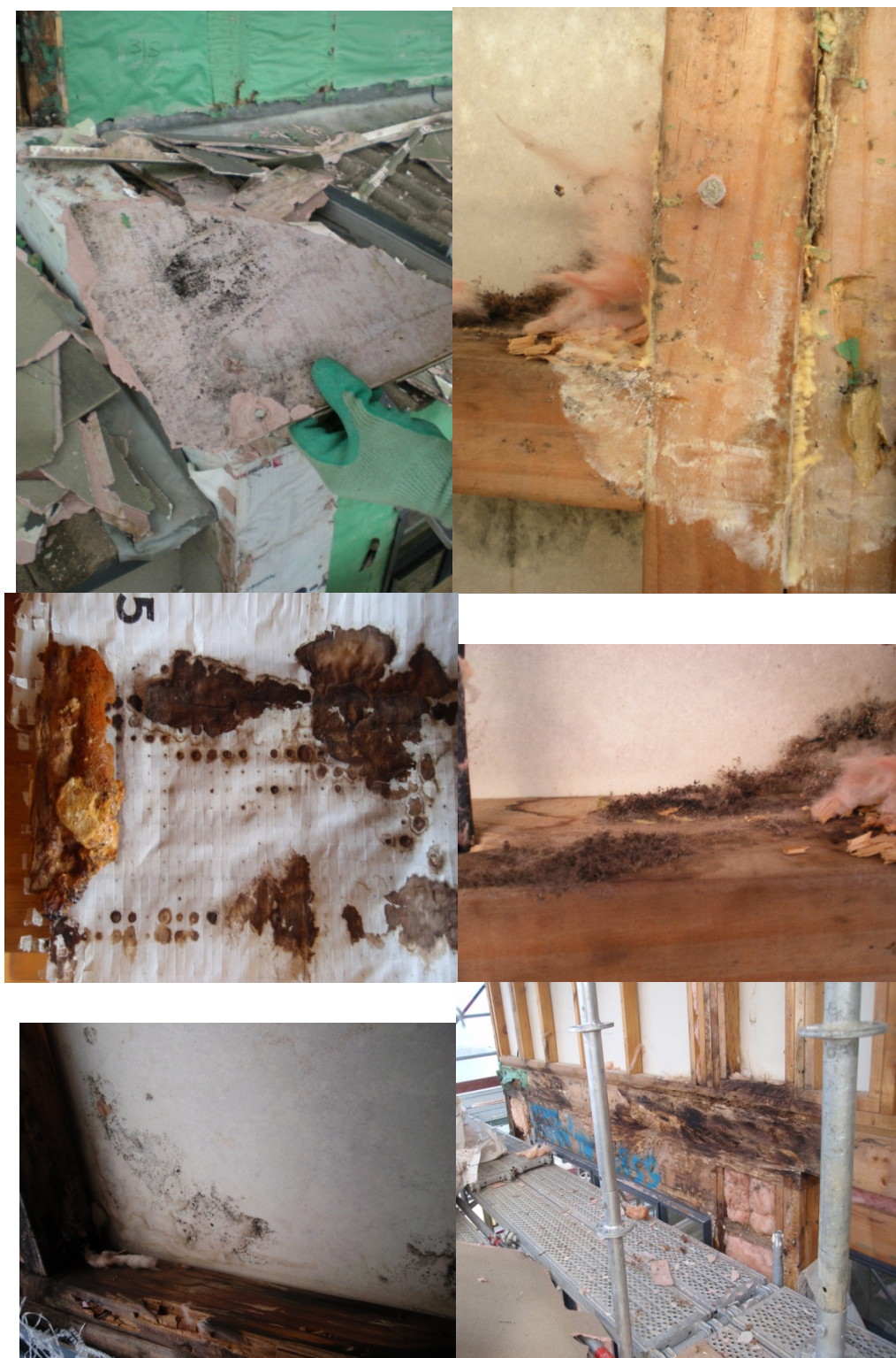
Figure 22: (Photo 17 – 22) All of the building materials damaged by water can support fungal and microbial growth. These pictures demonstrate fungal colonies seen on some of these materials.
