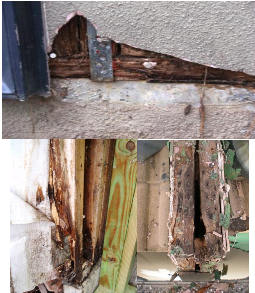
Figure 16: (Photo 8 – 10) Cladding removal also shows biodeterioration of the wooden structure of the Unit
