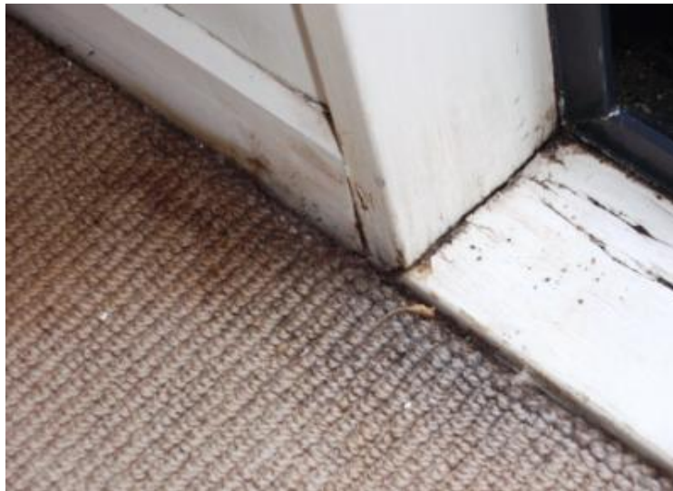
Figure 19: (Photo 14) Fungal contamination from water damage is also apparent on skirting boards and carpets.
