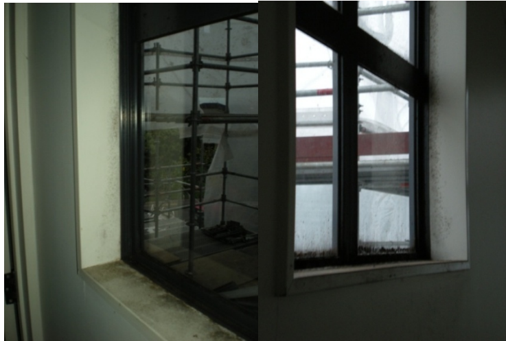
Figure 18: (Photo 12 & 13) Inside units fungal, biocontamination from water damage is apparent, particularly around windows
