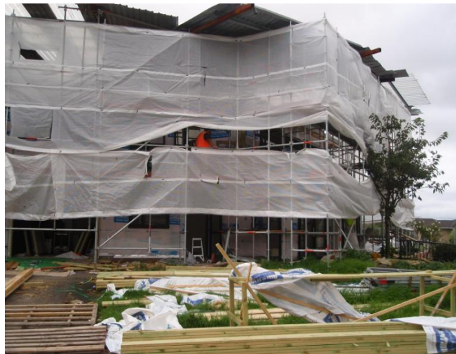
Figure 12: (Photo 2) Units during remediation phase in Complex 1 with scaffolding, temporary roof and screens attached
