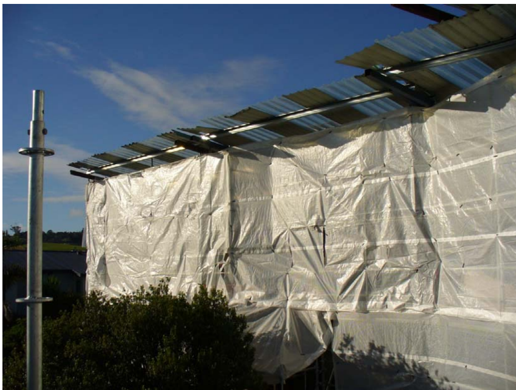
Figure 7: View of the temporary canopy of long run metal and translucent plastic sheets and plastic curtain surrounding the building being remediated
