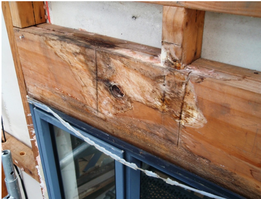
Figure 25: (Photo 25) Rhizomorphs of a basidiomycete wood decay fungus causing destructive brown rot on timber framing
