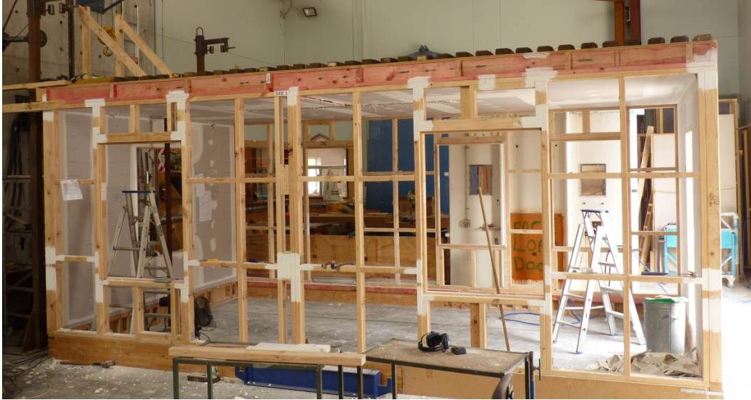
Figure 5 Construction for Phase 6
