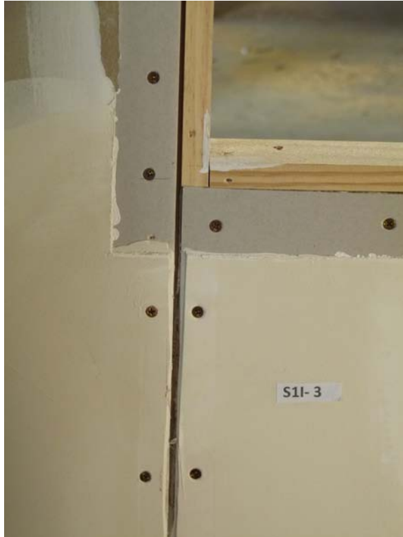
Photograph D15 taken during repair after Phase 3
