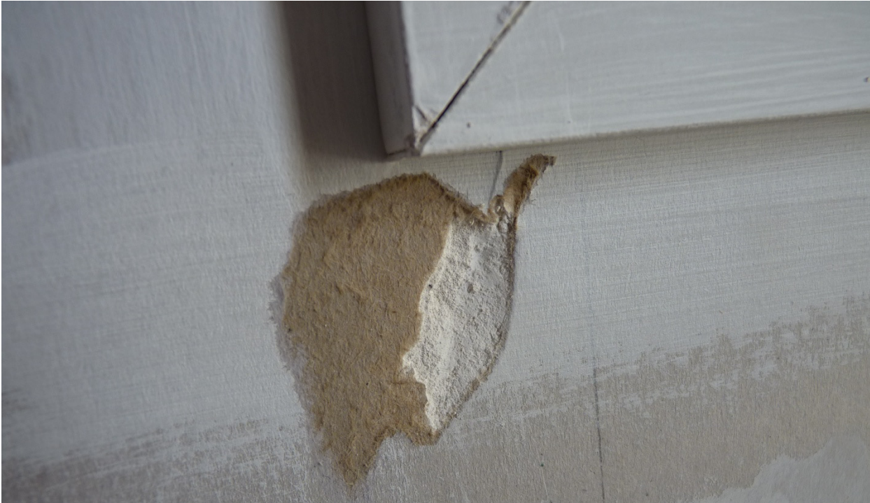
Photograph D5 cosmetic repair after Phase 1. Gouging out diagonal crack
