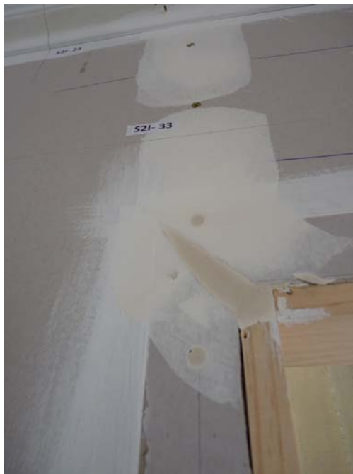
Photograph D18 during repair of a crack after Phase 3
