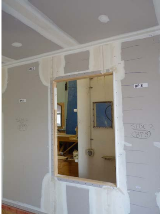
Photograph D19 taken during repair after Phase 3
