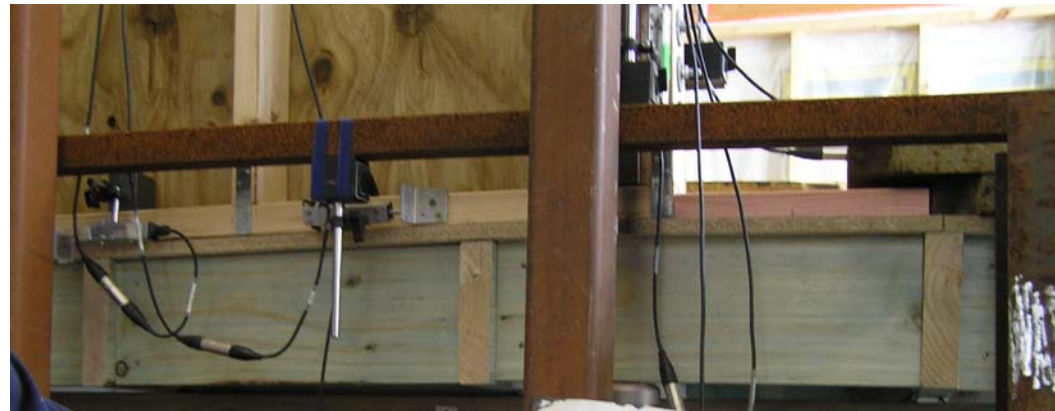
Figure 28. Test L1 – uplift at racking force = 8.42 kN pull at tension end of wall
