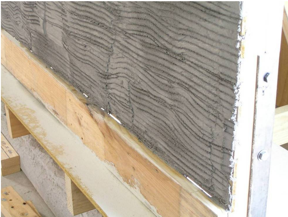
Figure 34: Scratched surface to receive second coat
