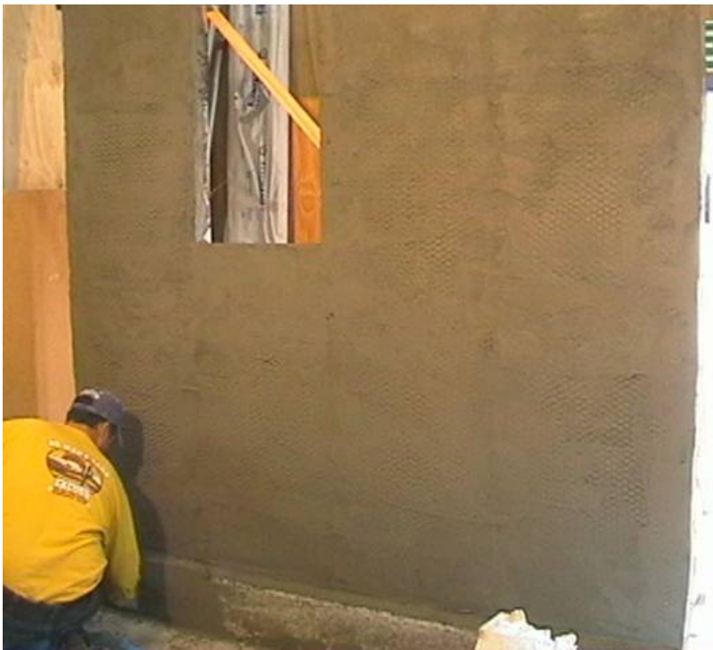
Figure 1: Building paper in place and chicken wire being added
