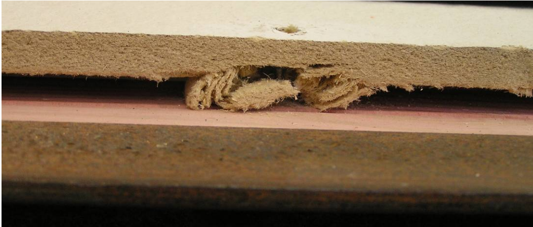
Figure 25: Damage to underside of softboard caused by movement with respect to nails
