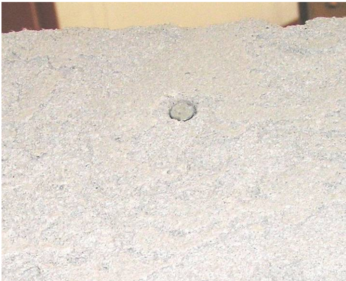
Figure 12: New nail added to re-attach the stucco panel to the framing (to be plastered)
