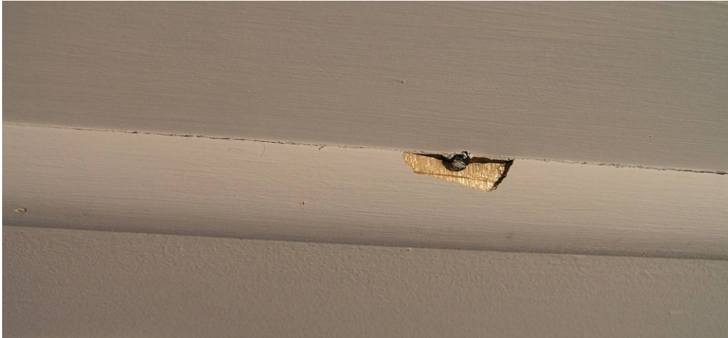
Figure 30: Damage to half round bead caused by panel pin head
