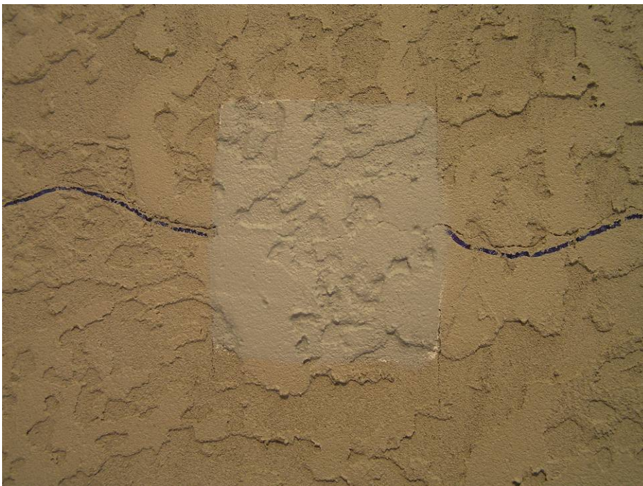
Figure 16: Crack after application of the top coat
