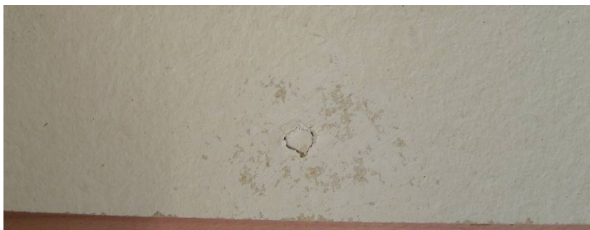
Figure 21: Nail head beginning to show through gypsum plaster
