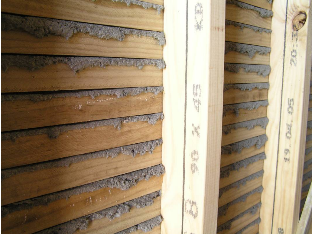
Figure 33: Plaster squeezed between the laths
