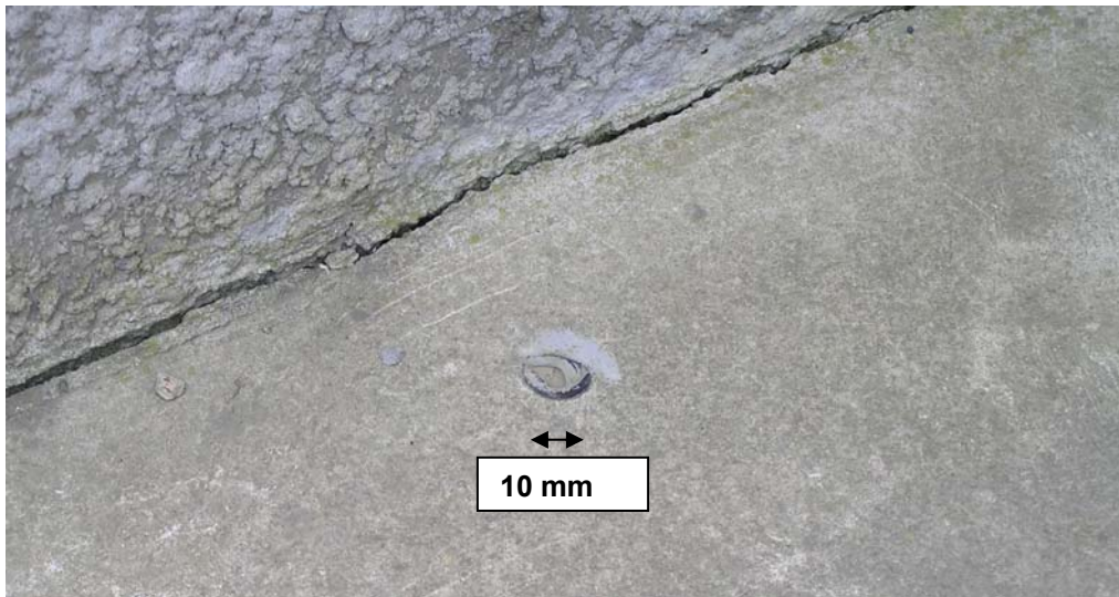
Figure 40: Evidence of the injection process beneath the yard slab
