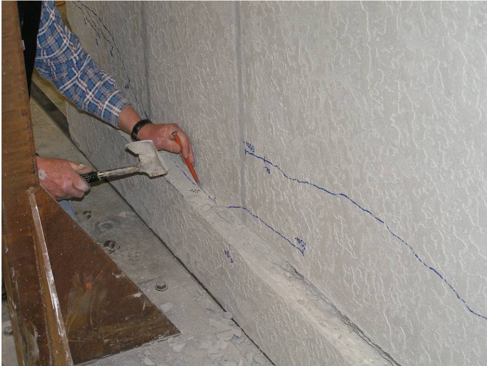
Figure 7: Removal of loose plaster at the foundation junction
