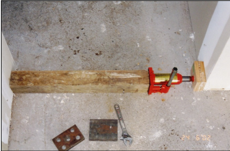
Figure 19: Car bottle jack used to translate the wall
