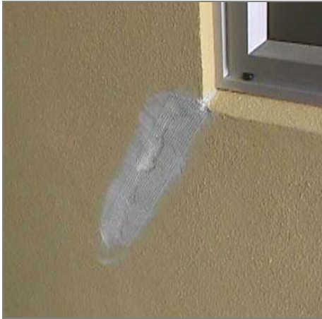
Figure 33: Crack in EIFS cladding prepared for filling
