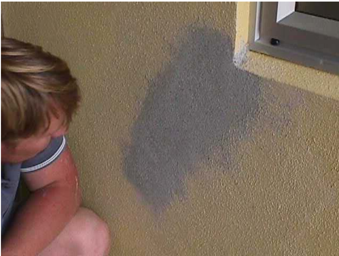
Figure 34: Feathering with a sponge to match the coating
