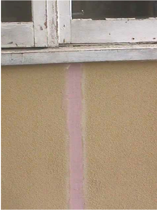
Figure 37: Fibre-cement joint filled with flexible jointing material
