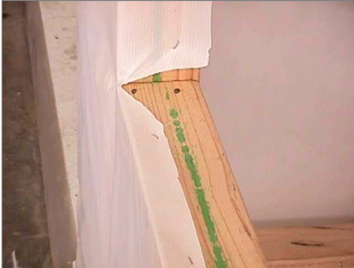
Figure 24: Building wrap mitred and fixed into the window frame
