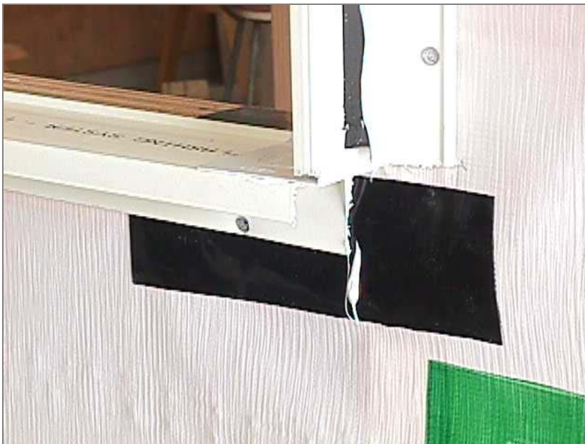
Figure 25: Proprietary flashings installed before the windows and EIFS cladding
