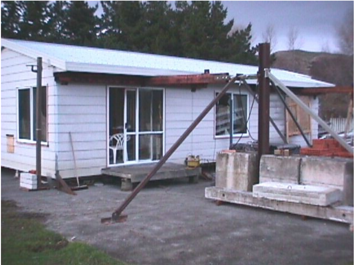
Figure 13: House to be plumbed (aligned vertically)
