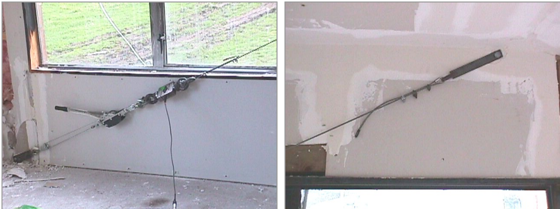
Figure 15: Light wire rope tensioning device and remote end connection
