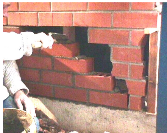
Figure 5: Replacement bricks being installed
