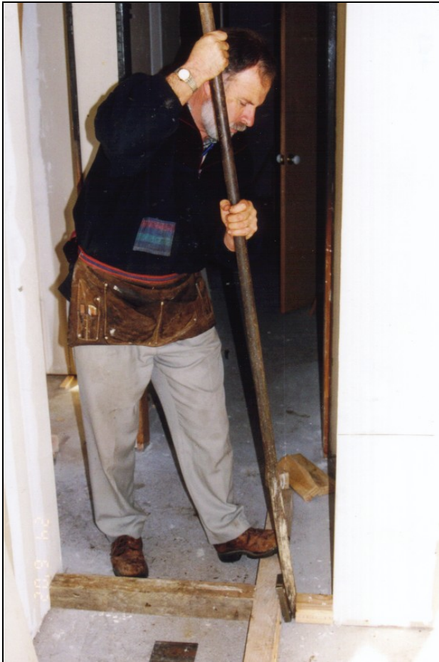
Figure 18: Re-aligning Wall 2 with a crow bar
