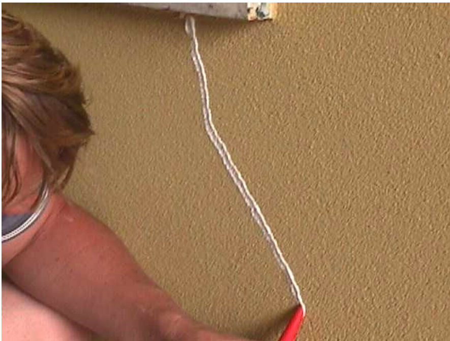
Figure 38: Filling the diagonal crack in the fibre-cement cladding with sealant
