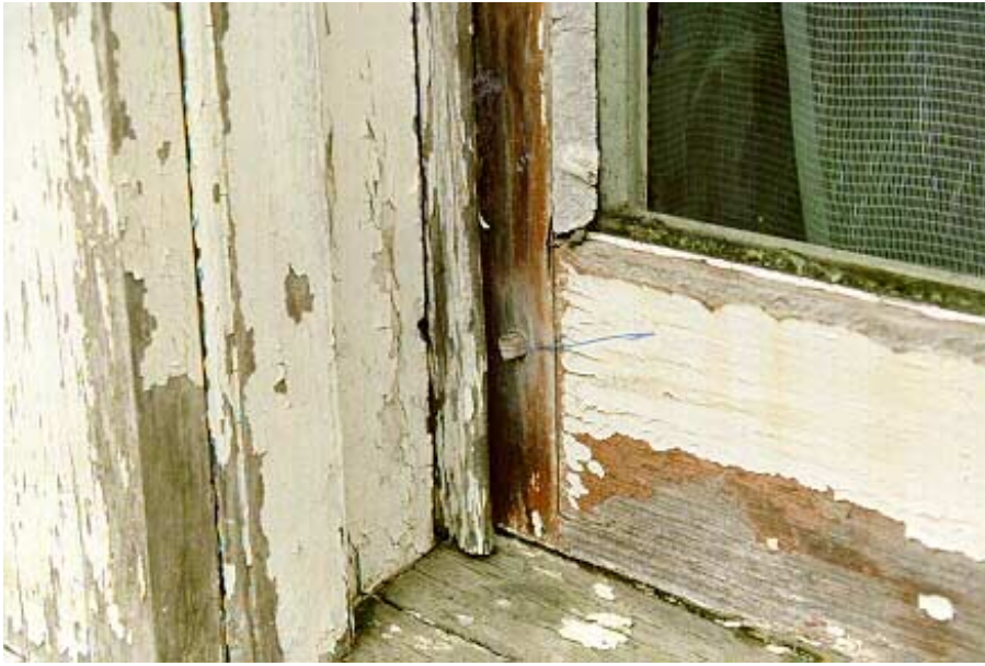
17 Above: Severe deterioration of paintwork in 1900's Auckland house. Note popping of dowel at joint, missing putty and splitting of timber.
