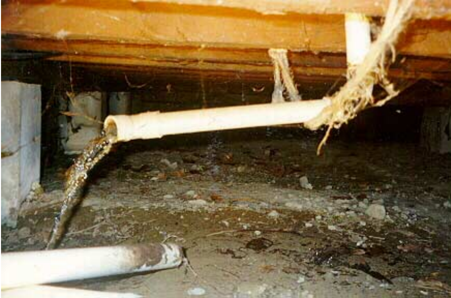
31 Above: Joint failure in PVC waste pipe allowing undetected discharge of wastewater into subfloor space (note pipe support).
