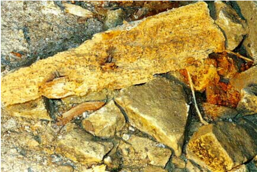
1 Above: Borer infestation in rubbish left in subfloor space. Also, high moisture levels in subfloor timbers from water seepage under house, and borer in floor joists.
