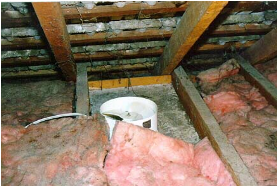
22 Above: Extractor fan discharging into roof space. Note insulation not replaced after installation.
