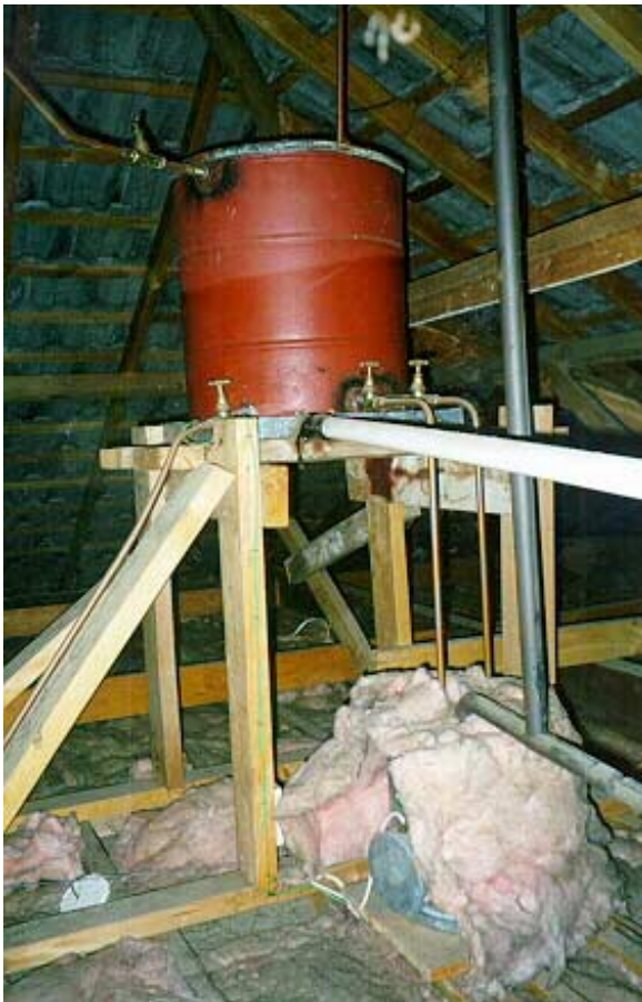
29 Above: Heavy concrete header tank not restrained against earthquake movement (note also the state of the pipe lagging and ceiling insulation).
