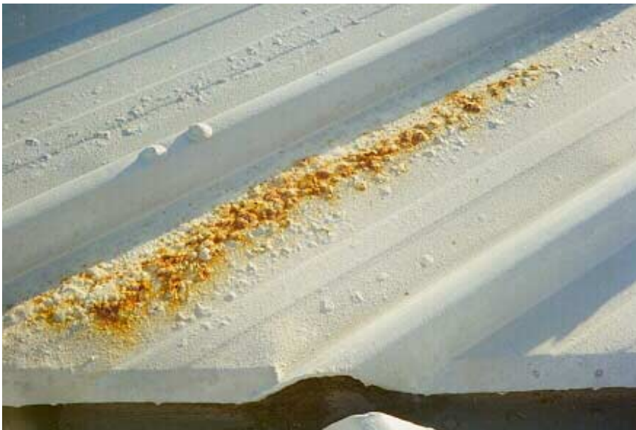
40 Above: Severe corrosion to longrun galvanised steel roofing in 1980's Wellington house (exposed to severe marine environment).
