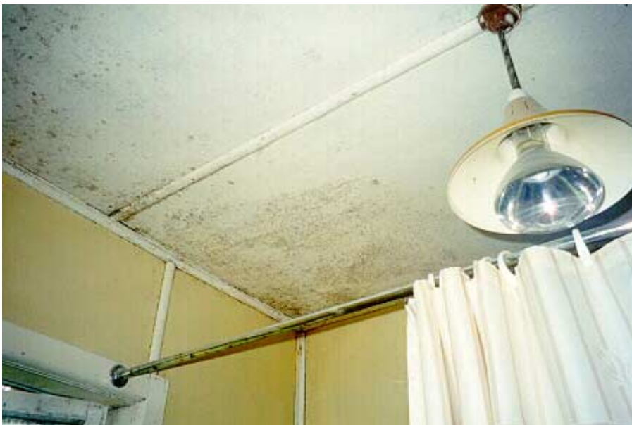
45 Above: Lack of bathroom ventilation causing high levels of mould and mildew on painted hardboard linings.
