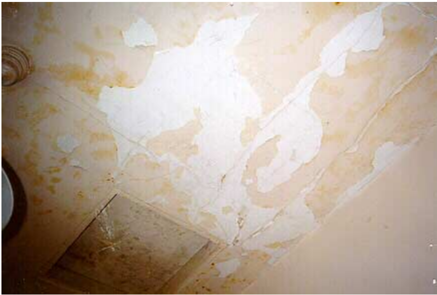
46 Above: Extreme levels of mould and mildew on lathe and plaster linings to 1920's Auckland house (same house as in photograph 18).
