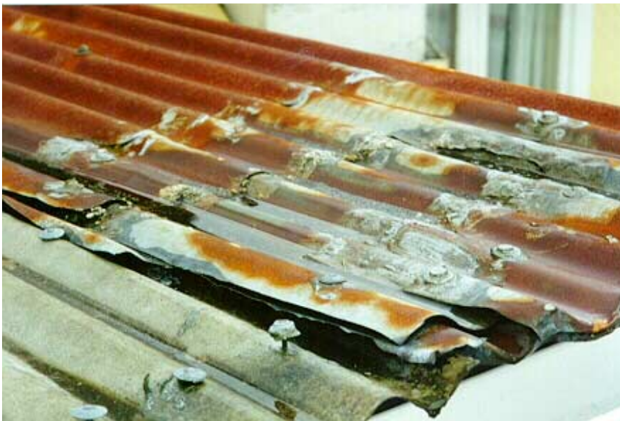
38 Above: Severe corrosion to old galvanised steel roof in Wellington house (note: same house as shown in photograph 35).
