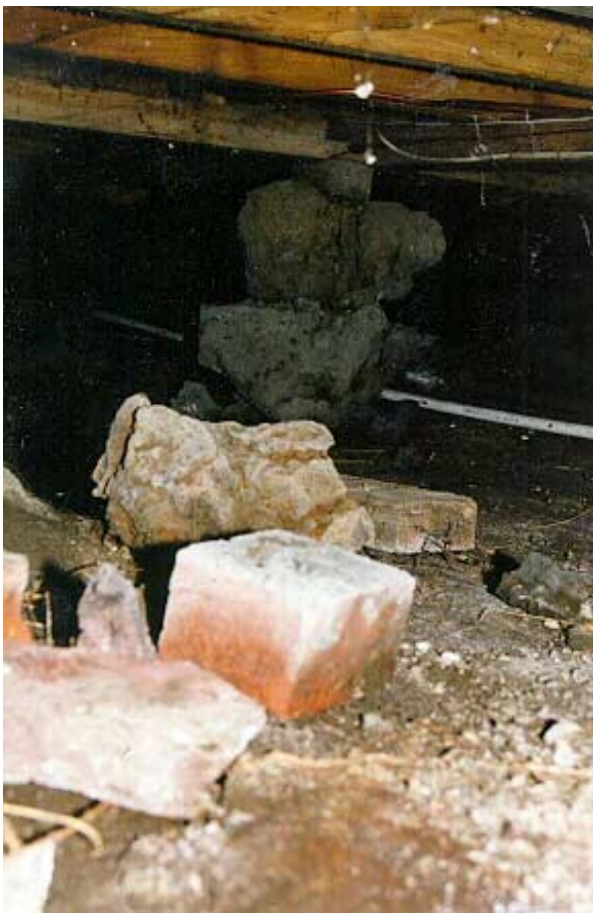
12 Left: Seventy year old Auckland house with stacked rocks as supports to floor joists (along with a variety of other types).
