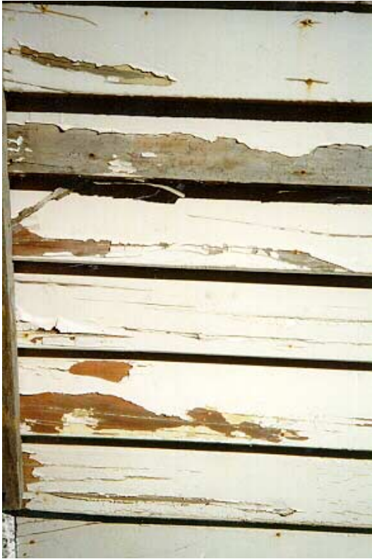
15 Left: Deterioration of paintwork on 1930's Christchurch house. Cladding has rusting nails, major splitting of boards and severe borer.
