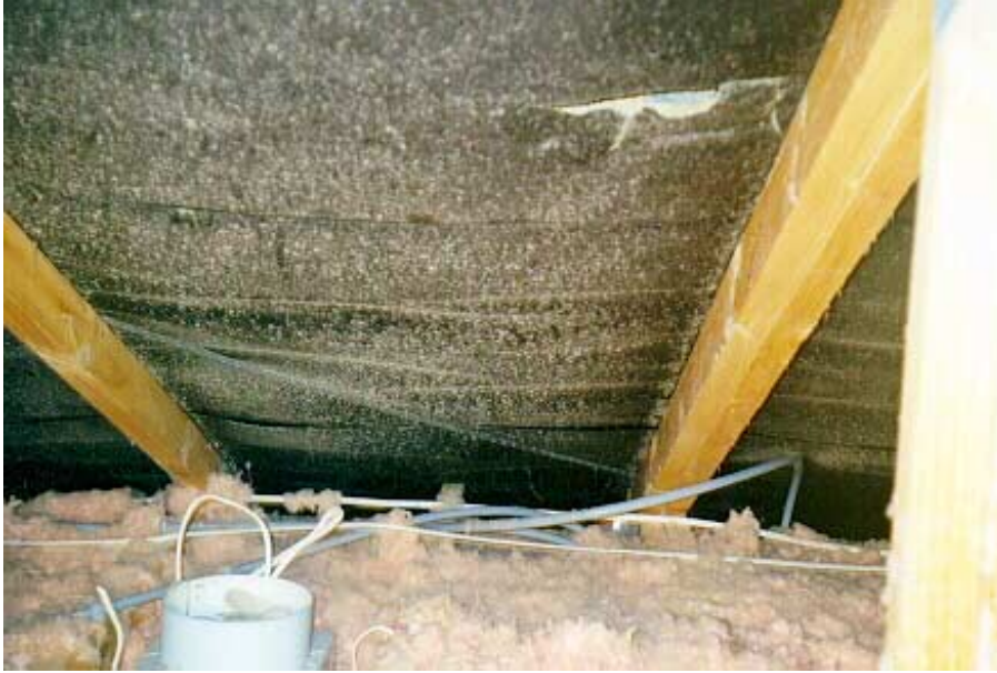
21 Above: Bathroom extractor fan discharging into roof space. Note damage to building paper above fan.
