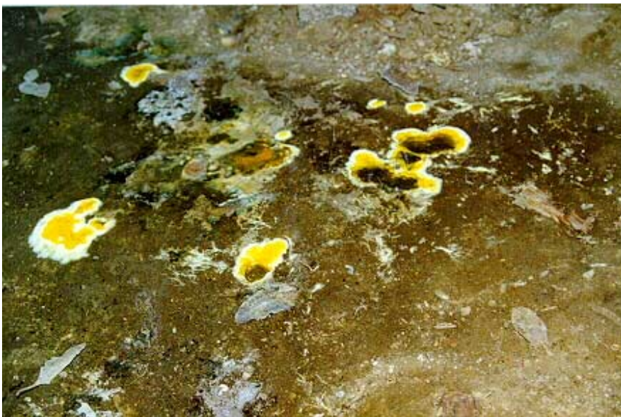
2 Above: 1960's house which felt damp inside. Fungal growth on soil under house indicating high moisture levels. House also had sub-standard subfloor ventilation, with some vents blocked off as shown in photograph 13.
