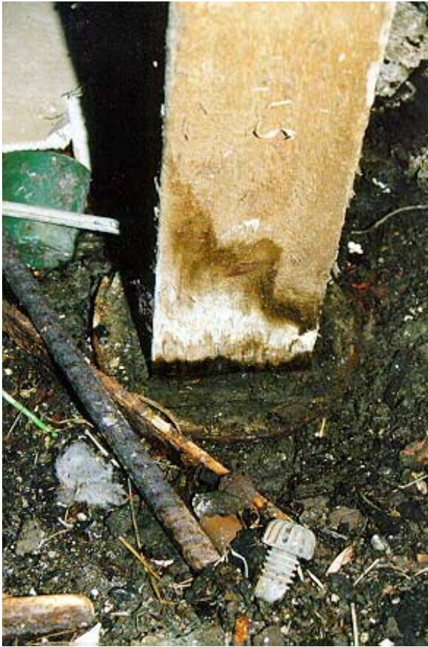
3 Left: Timber pile showing water stains. Concrete pile is level with surrounding soil.
