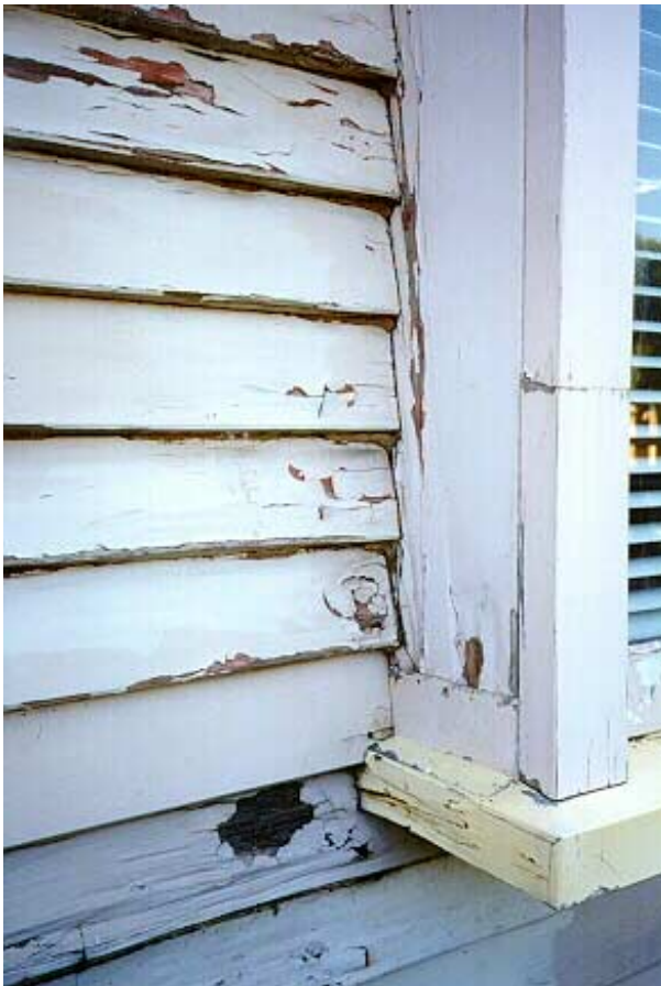
17 Above: Severe deterioration of paintwork in 1900's Auckland house. Note popping of dowel at joint, missing putty and splitting of timber.
