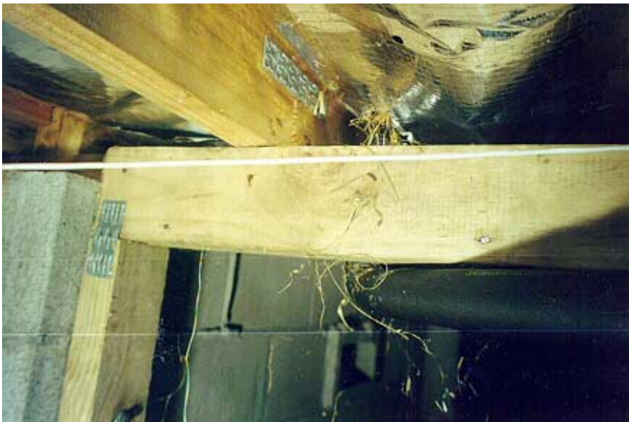
10 Above: Rats' nesting in drooped foil insulation (beneath hot water cylinder).
