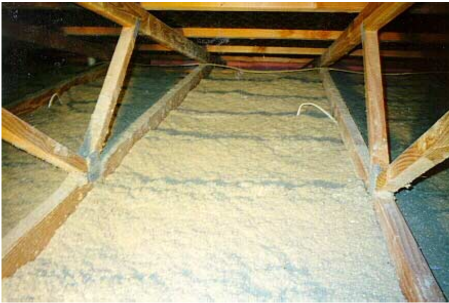
25 Above: Loose fill macerated paper insulation settling with age and deteriorating in efficiency (average thickness is now less than 50mm)
