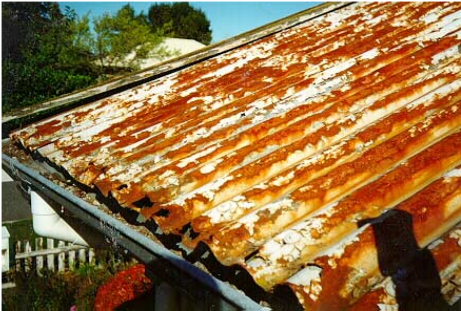
37 Above: Severe corrosion to old galvanised steel roof in Auckland house (note: same house as shown in photograph 18).
