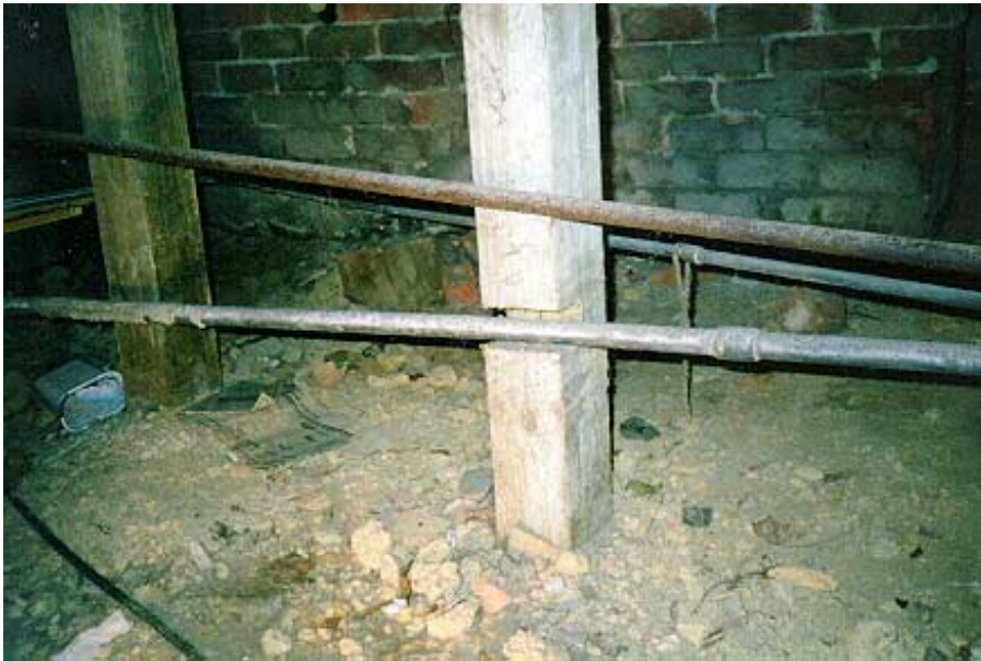
11 Above: Old timber jack stud rebated for water pipe.
