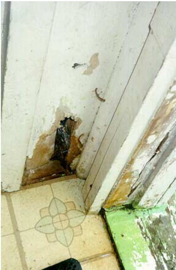
47 Left: Poor condition of exterior shell causing decay visible inside the 1940's Wellington house (same house as in photograph 39).
