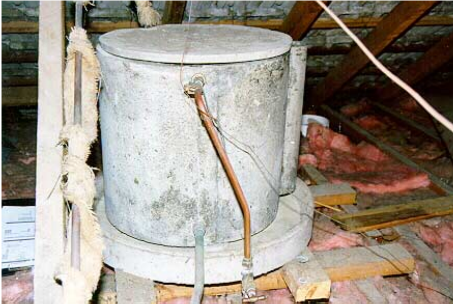
29 Above: Heavy concrete header tank not restrained against earthquake movement (note also the state of the pipe lagging and ceiling insulation).
