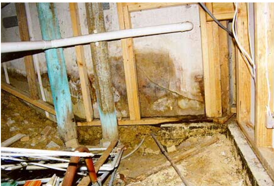
4 Below: Decay in bottom wall plate and moisture damage to back of basements linings. Large 1980's Auckland house. No subfloor ventilation and high moisture levels.
