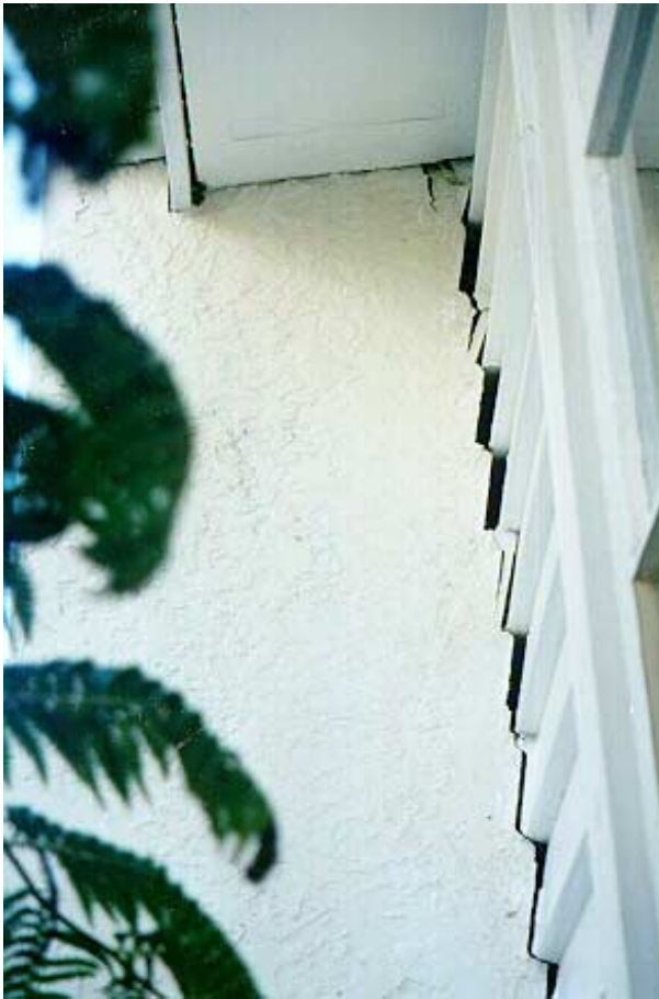
19 Left: Crack showing movement of chimney away from timber wall.
