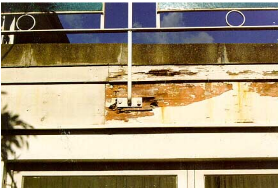
20 Below: Severe decay endangering fixing of handrail support.
