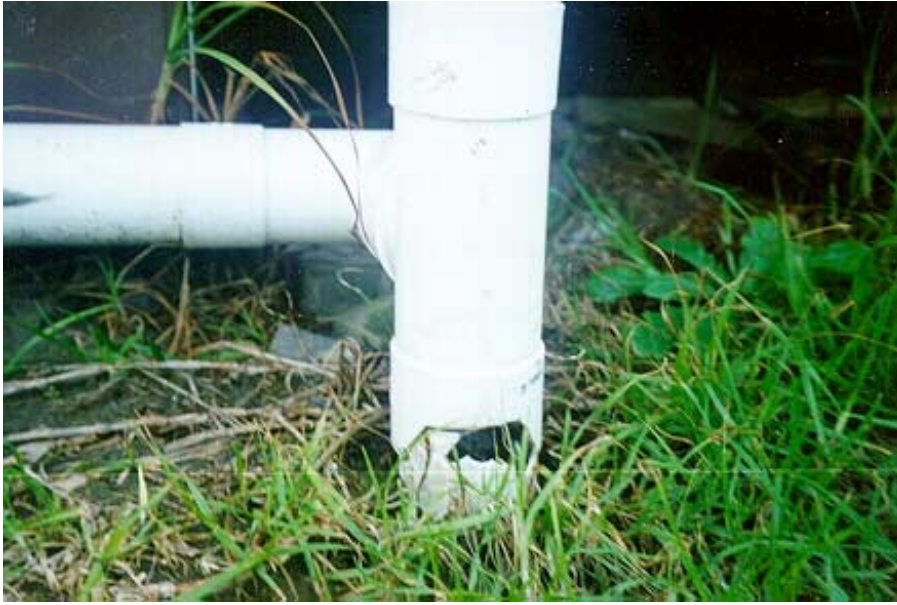
43 Above: Damaged PVC downpipe allowing stormwater discharge onto soil and subsequent moisture problems in adjacent subfloor space.
