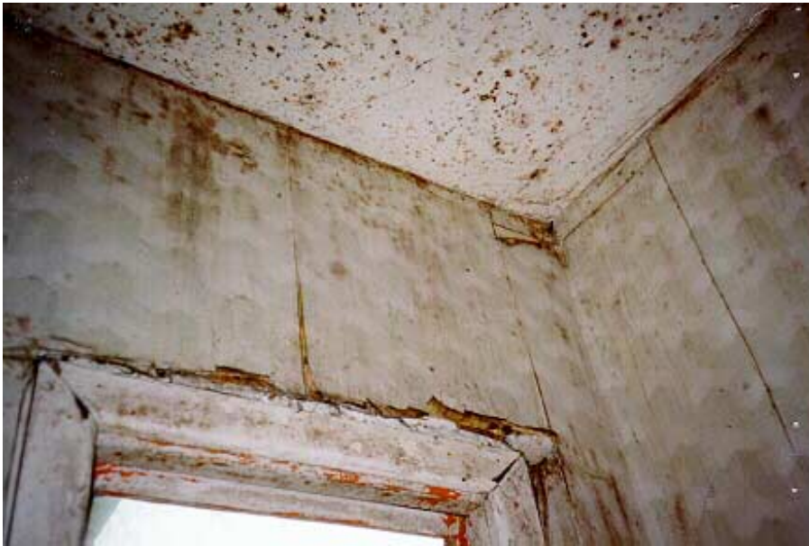
44 Above: Extreme levels of mould and mildew on lathe and plaster linings to bathroom of 1900's Christchurch house (same house as in photograph 16).
