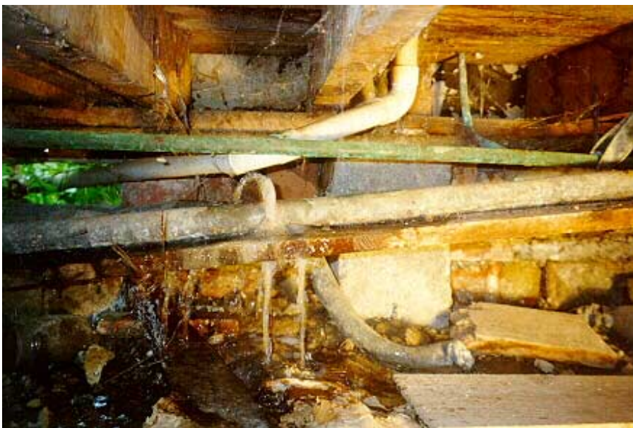
34 Below: Deterioration in 60 year old lead waste pipes lead to undetected discharge into subfloor space. Unable to detect how long pipe had been leaking, but moisture levels were high and the native timbers were heavily infested with borer.
