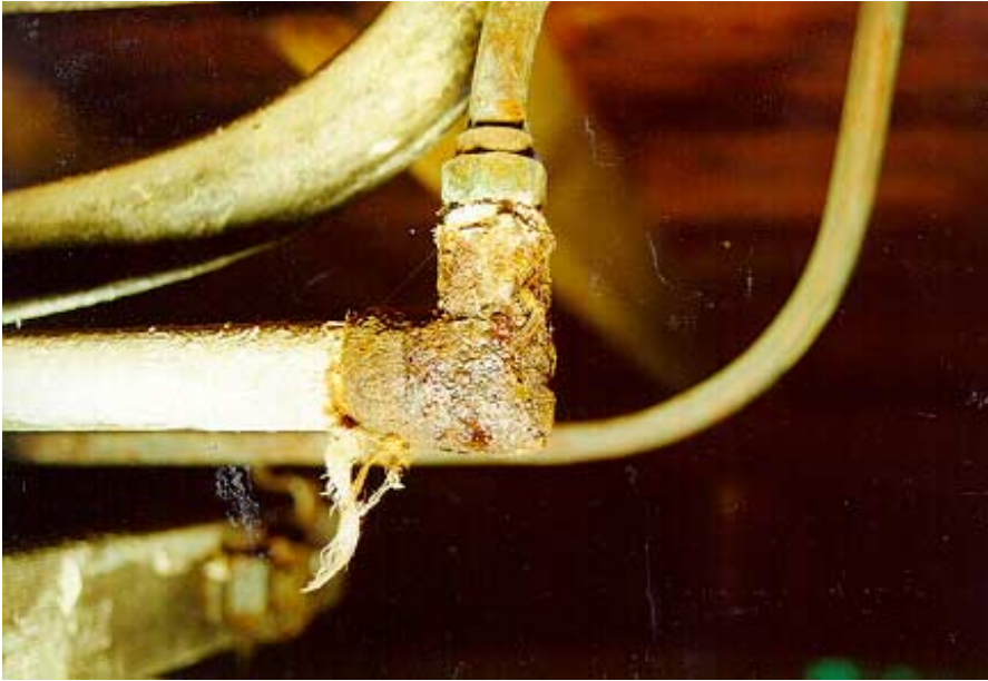
35 Above: Corrosion in joint of galvanised steel water pipe likely to cause a leak.
