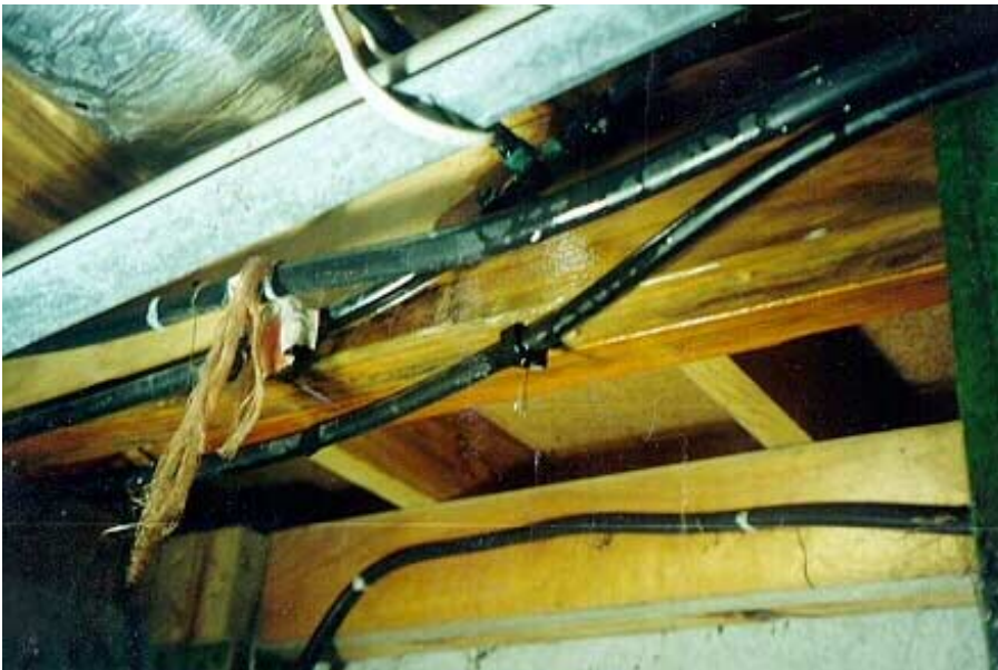
36 Above: Joint failure in polybutylene hot water supply pipework (note drips and wet timber).
