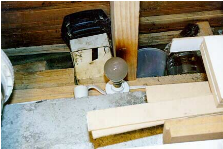
23 Above: Light fitting installed too close to timber causing a fire hazard. Note scorching of timber and paint materials stored alongside light.
