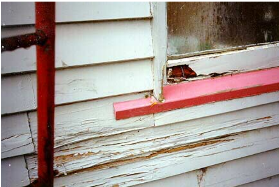
16 Below: Severe decay in weatherboards and windows in 1900's Christchurch house.
