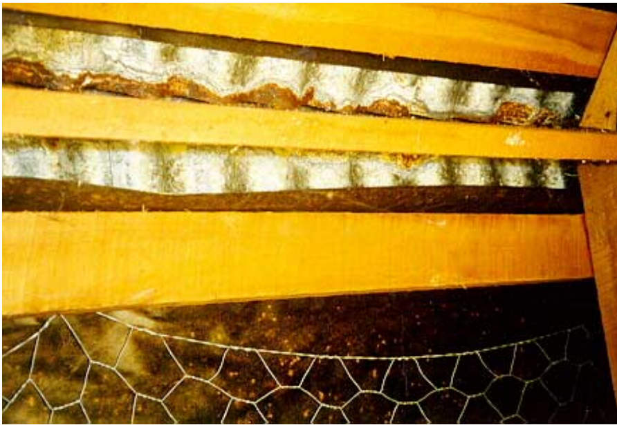
39 Above: Faulty ridge flashing leading to corrosion.
