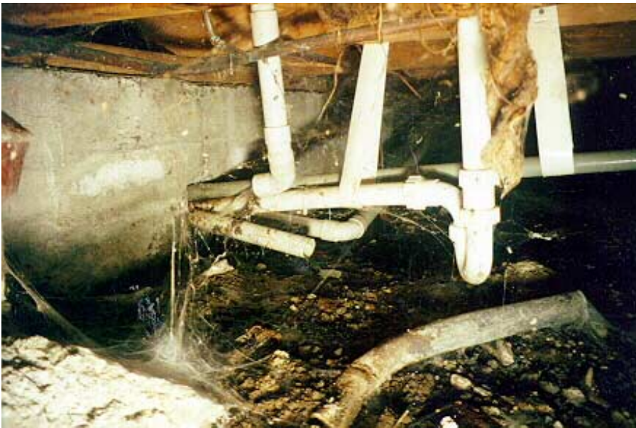
32 Above: Joint failure in PVC waste pipe allowing undetected discharge of wastewater into subfloor space (note also state of hot water pipe lagging).
