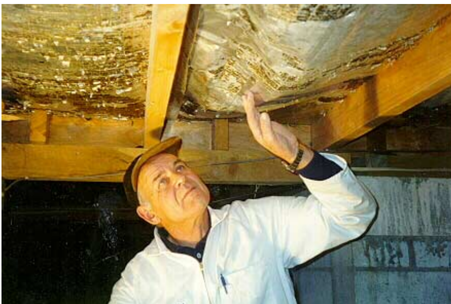
8 Below: Underfloor foil insulation degrading. 1980's house exposed to severe marine environment.
