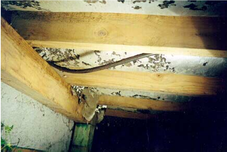
9 Above: Same house as shown in photograph 6. Breakdown of foil backing to particleboard flooring in house in severe marine environment (with sufficient subfloor ventilation).
