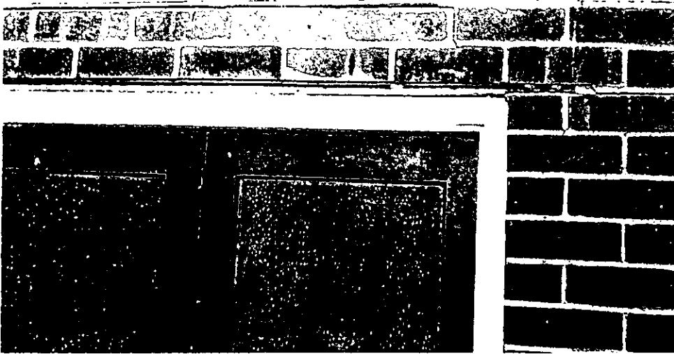
Brick lintel cracks.
