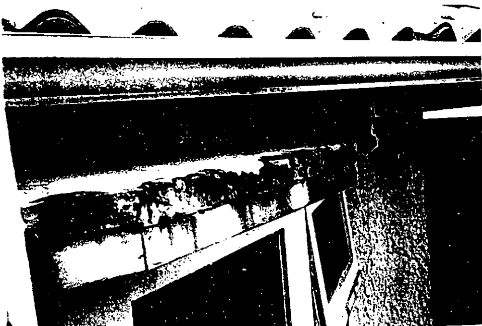
Serious corrosion in window head flashings.
