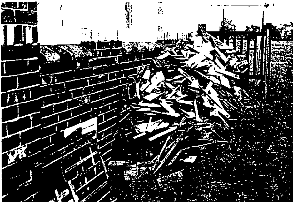
Firewood blocking sub- floor vents.
