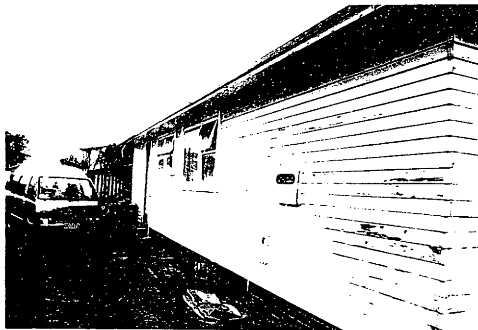
TOP & MIDDLE. Paint deterioration to bare timber.
