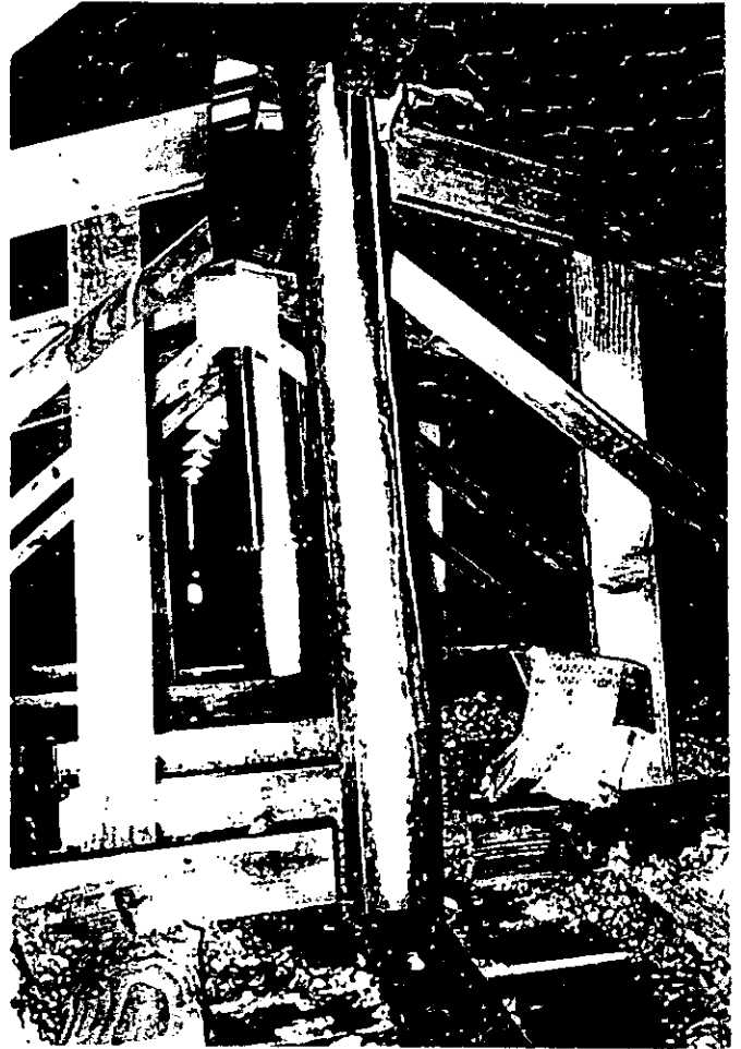
TOP LEFT. Unsafe support to the header tank.
