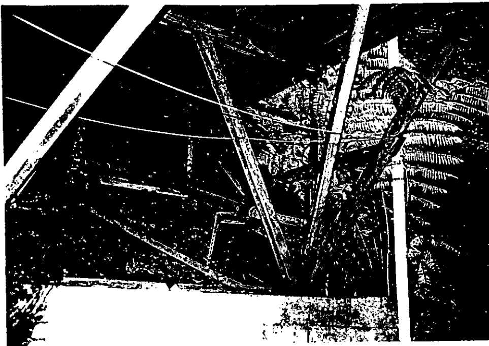
Inadequate connections to the foundation and bearers.
