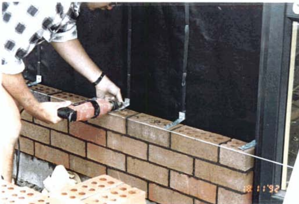
Photograph 14: Installing ties using screwdriver
