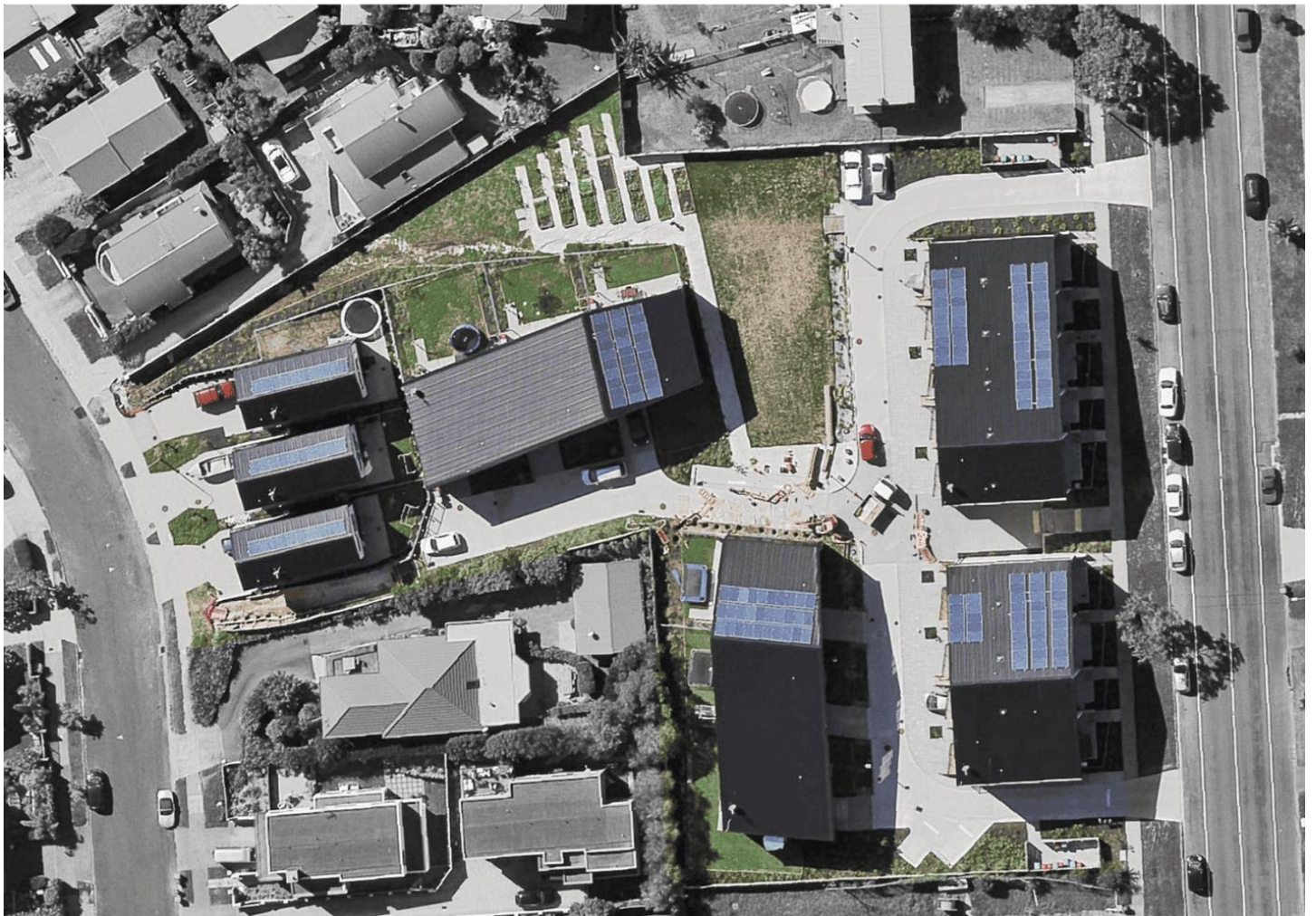
ABOVE: Leasehold subdivision plan (top) and aerial photo (bottom) of part of the kāinga (18 of the 30 homes). Private lease areas are shown white on the leasehold plans, corresponding to the 150-year leases each whānau have to the land on which their home sits.
