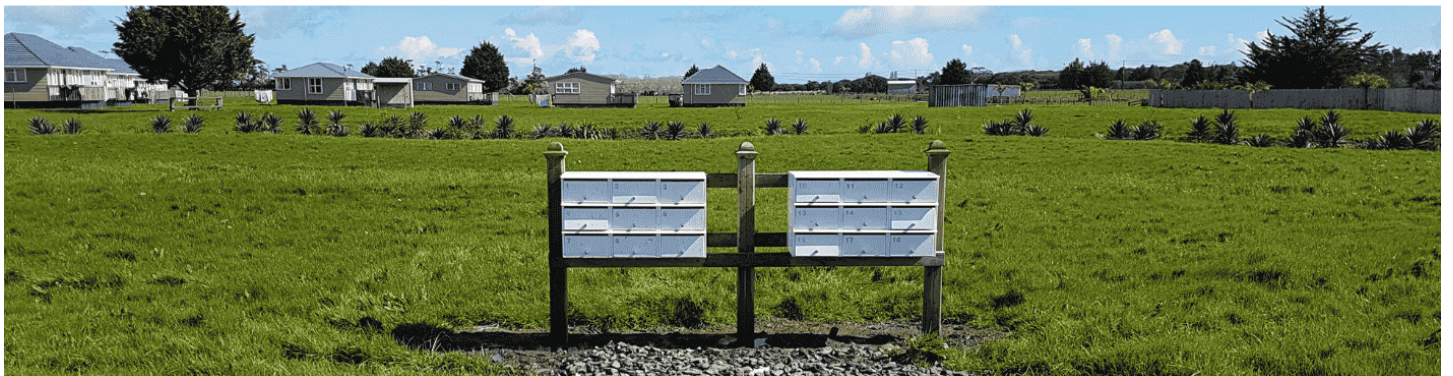
ABOVE: Images of He Korowai Trust's kāinga shortly after the completion of Stage 1 (9 houses) on site in 2017, with relocated and refurbished ex-Kāinga Ora state houses on the site, as well as extensive stormwater management (swales and open green space).
