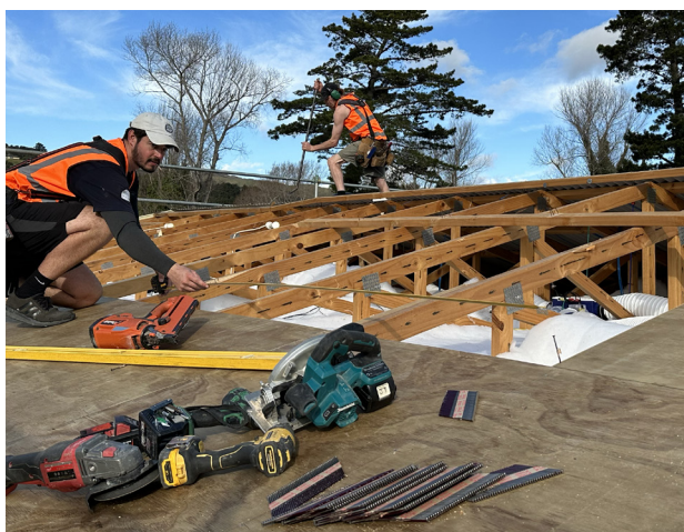
Figure 3. The plywood substrate being installed for the warm roof on the BRANZ ventilation test building.
