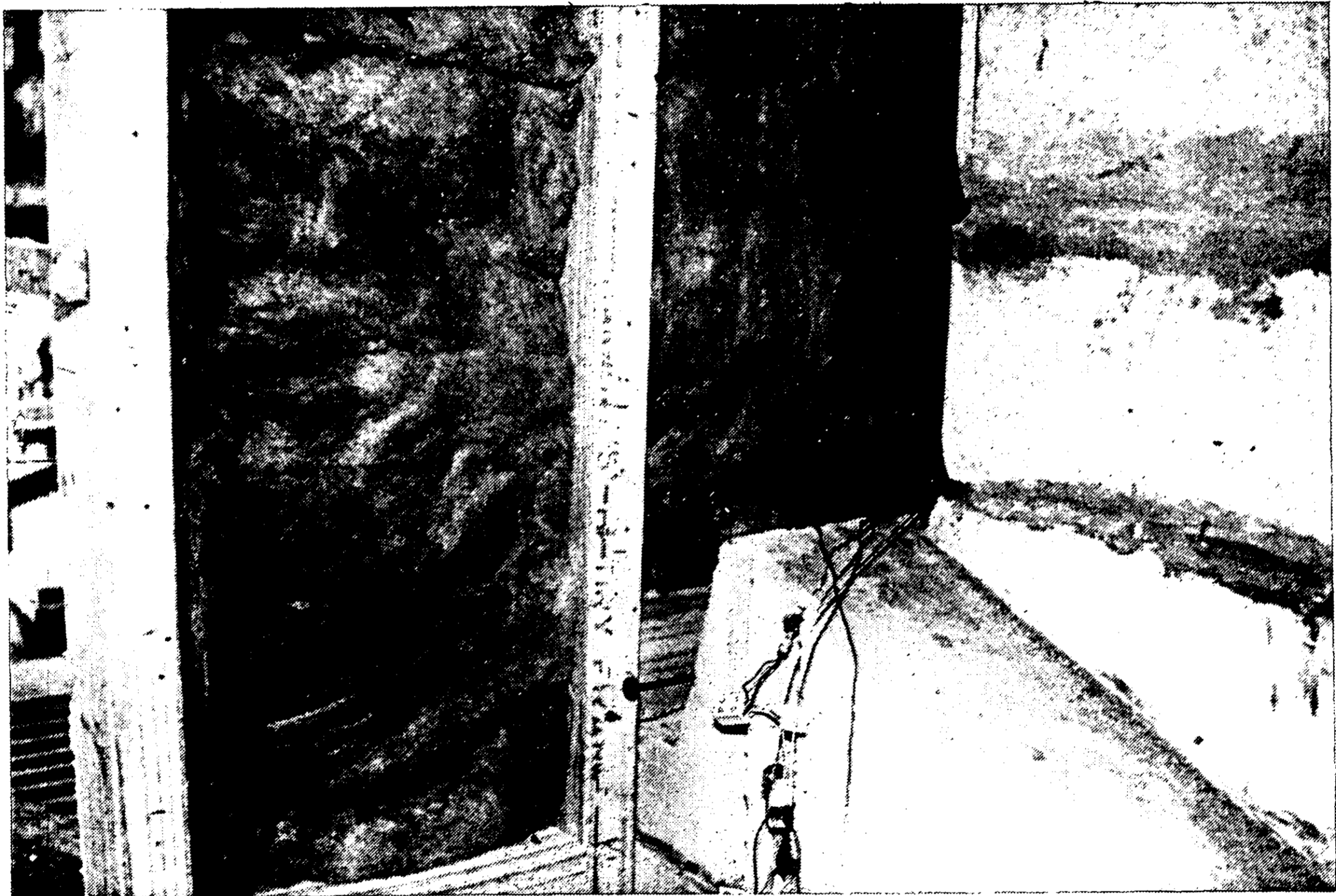
Figure 6: Test rig detail prior to weatherboard installation.
