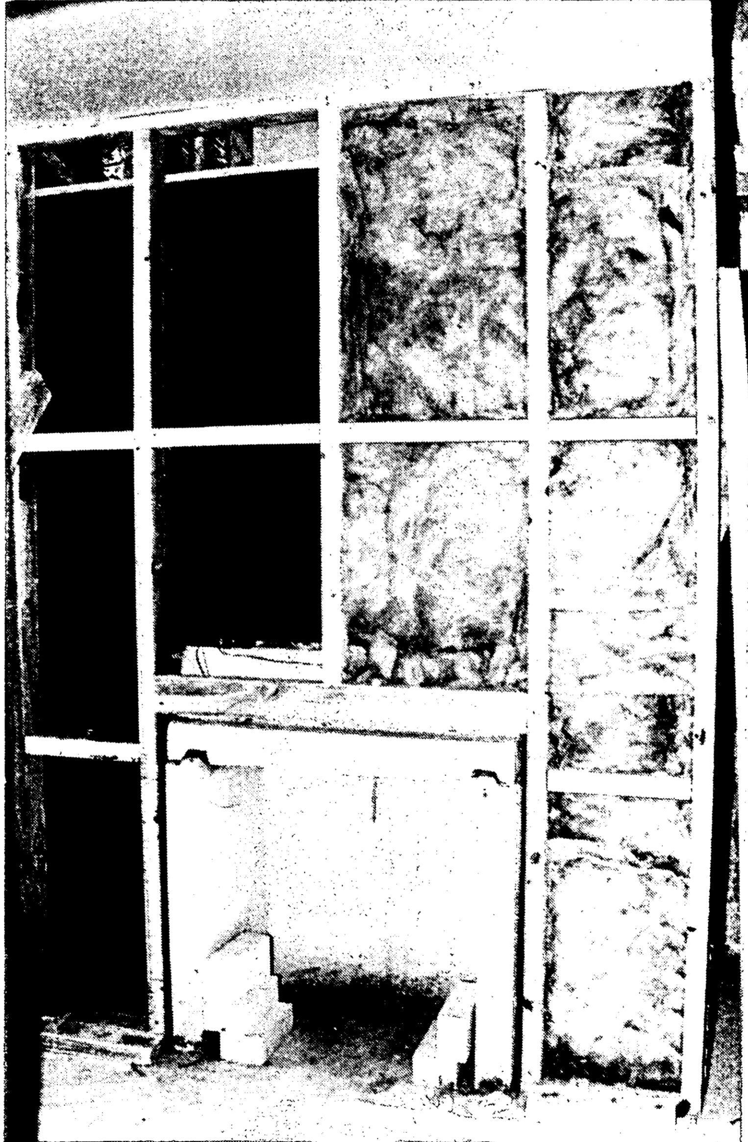
Figure 4: Test rig during construction, with framing at 25 mm clearances.
