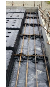
Figure 12 - Reinforcing bars on the CLEVA POD® spacers™. (Clevaco, 2022).
