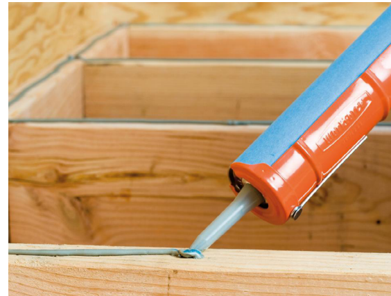
Figure 25 - Adhesive applied to floor joists. (ConstructionMentor.net, n.d.)
