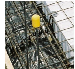
Figure 6 - RibRaft installation closeup. (Firth Industries, 2023).
