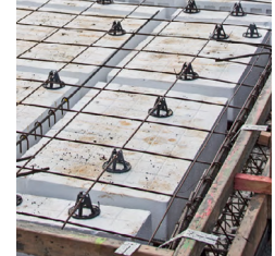
Figure 5 - Rebar chairs in the RibRaft System. (Firth Industries, 2019).
