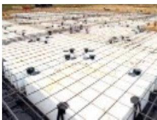
Figure 9 - RibRaft installation. (Firth Industries, 2012).
