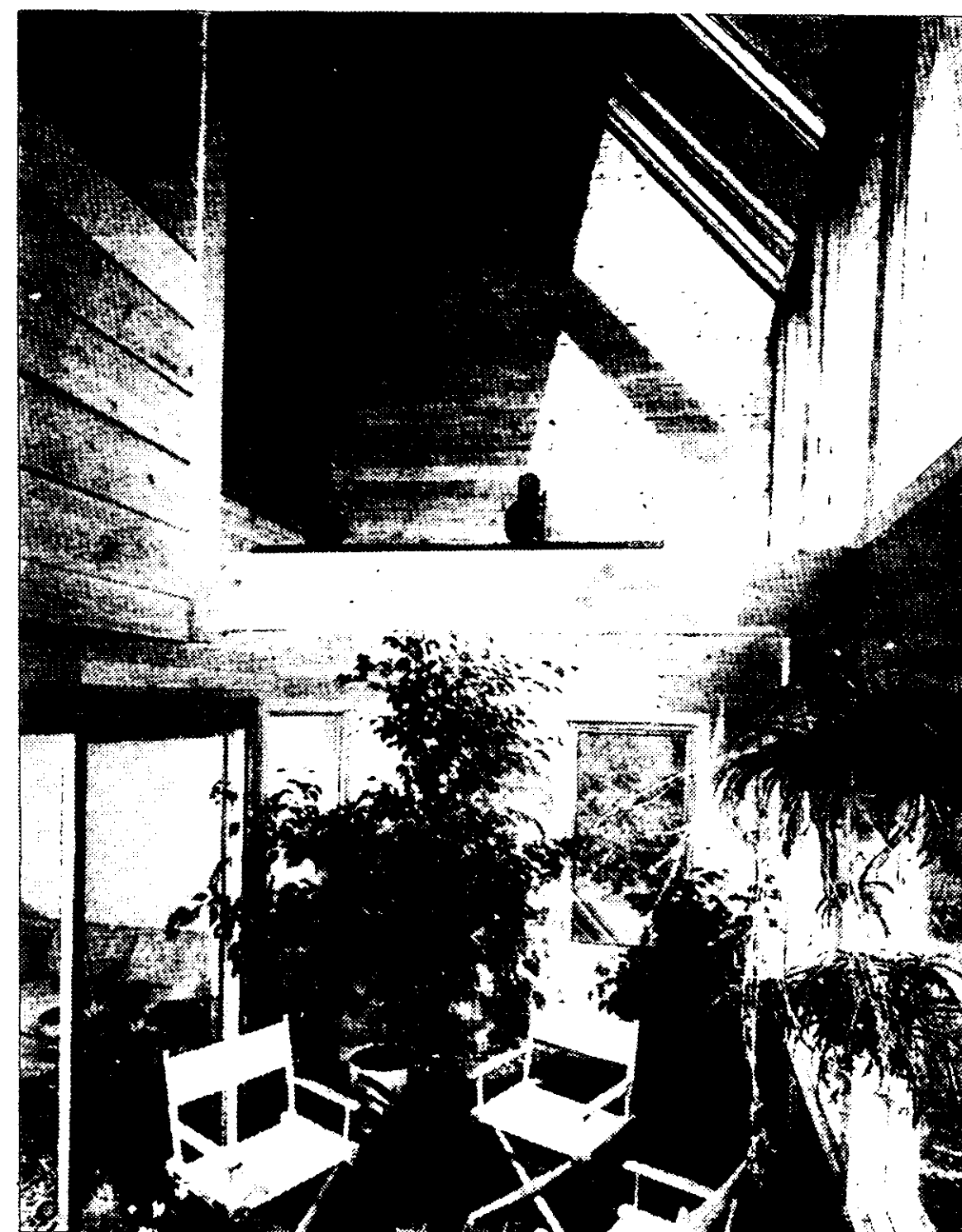
Isolated gain sunspace is closed off from the house.
