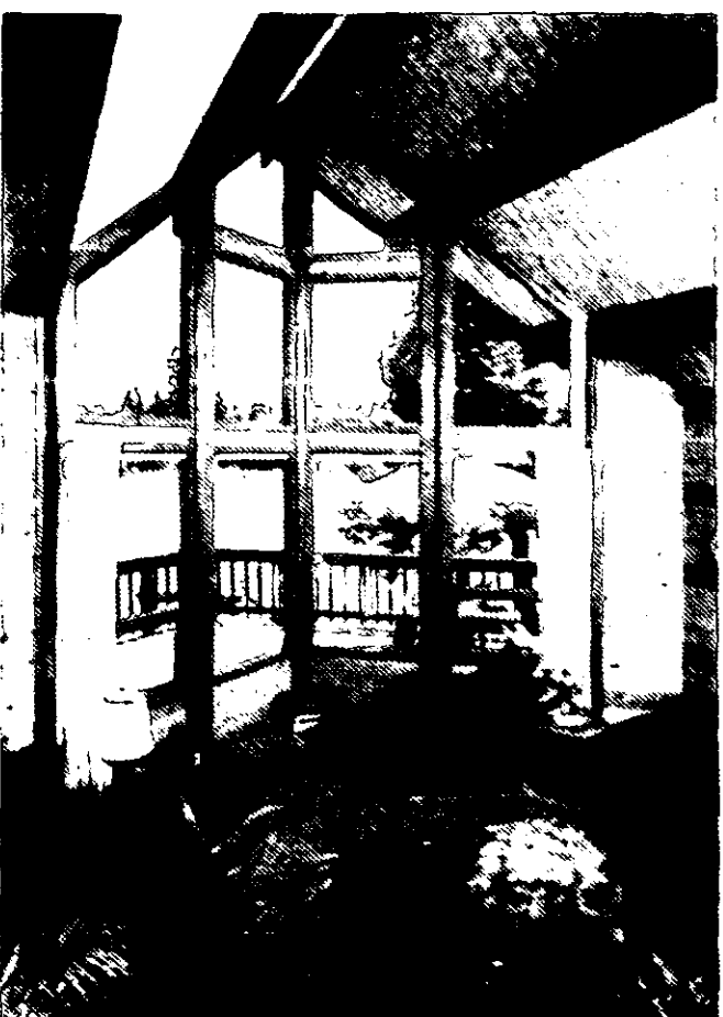
Justus: Single wall, solid wood construction. The outside walls are constructed of solid, four-inch thick cedar timbers positioned horizontally. Inside, partitions are drywall with cedar timbers an option.
