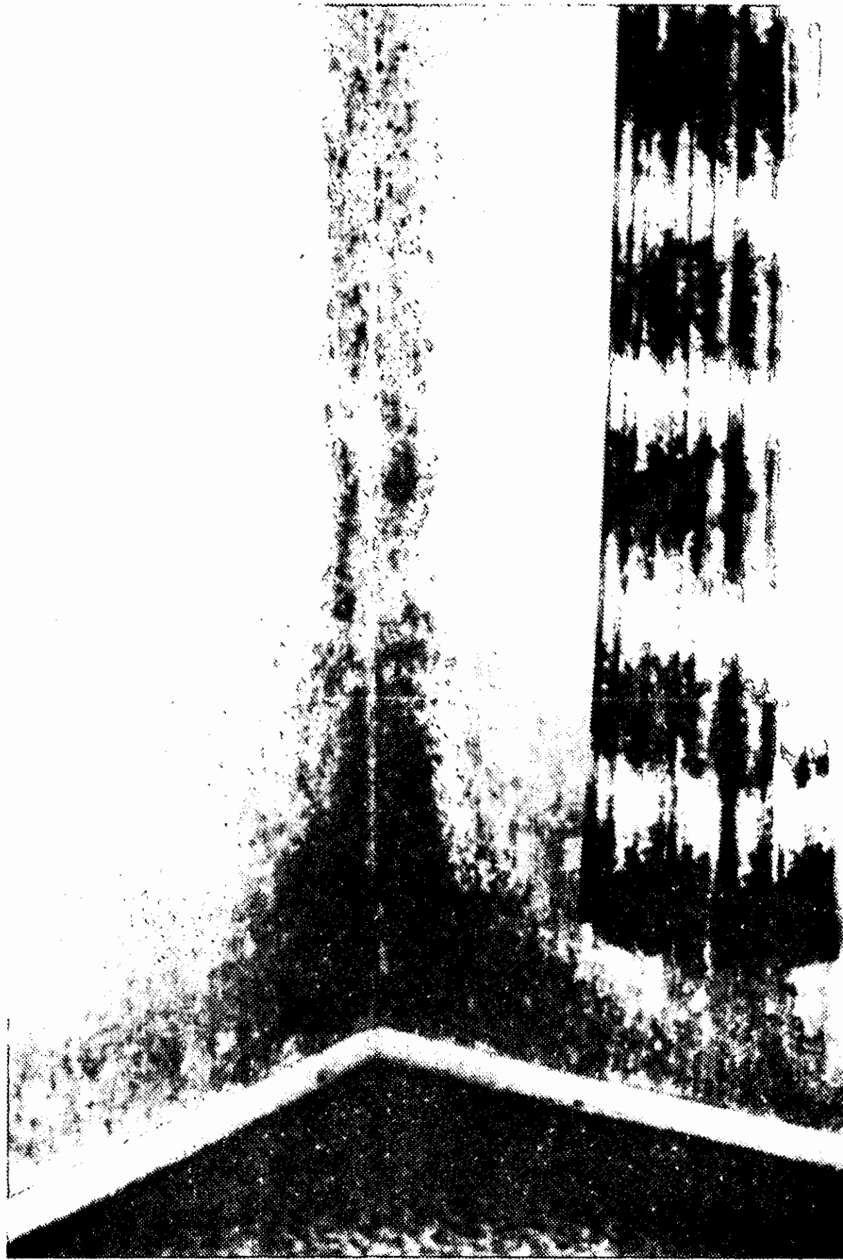
Figure 2 : Mould growth near corner due to inadequate wall insulation.
