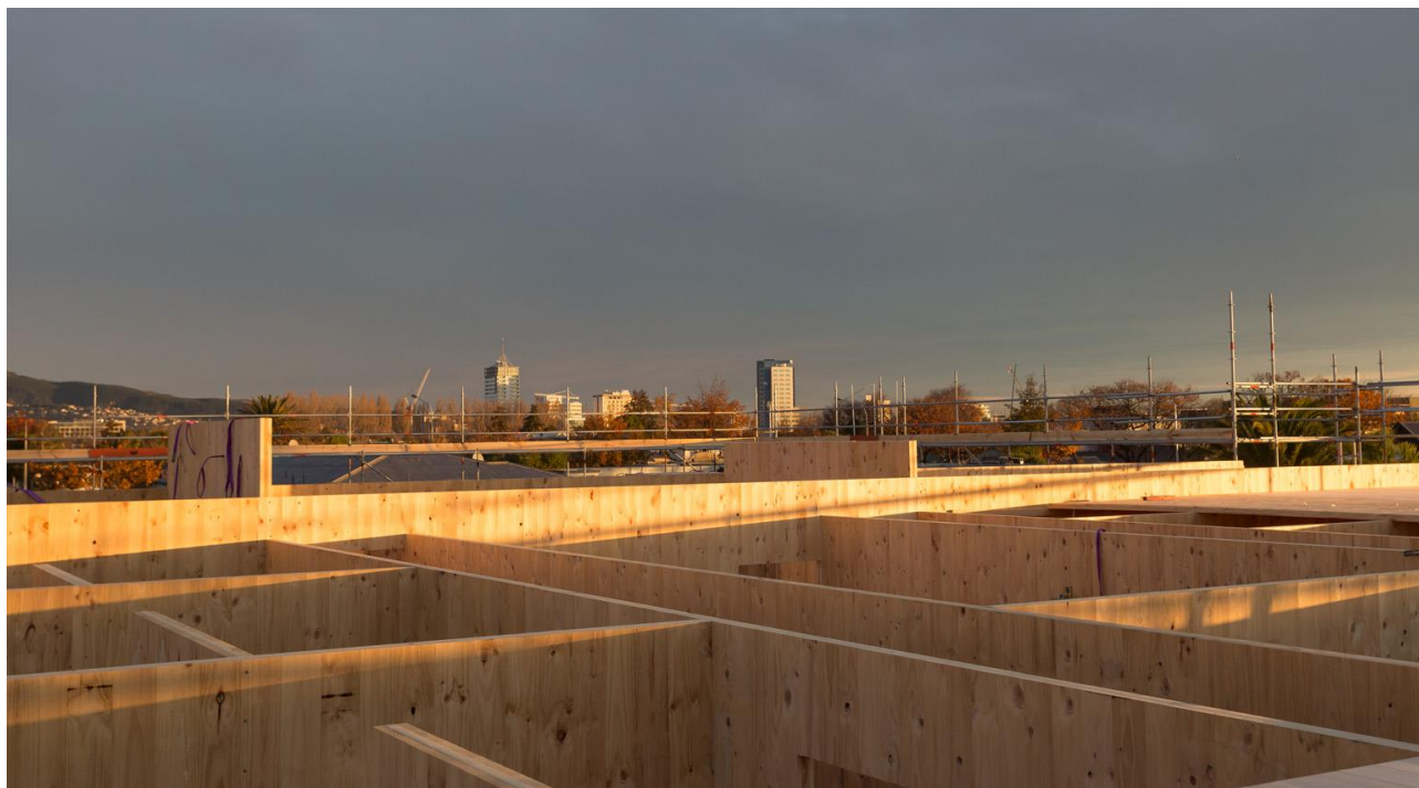
Figure 9 Distributed lateral systems on display at Bealey Lodge (courtesy of EngCo)
