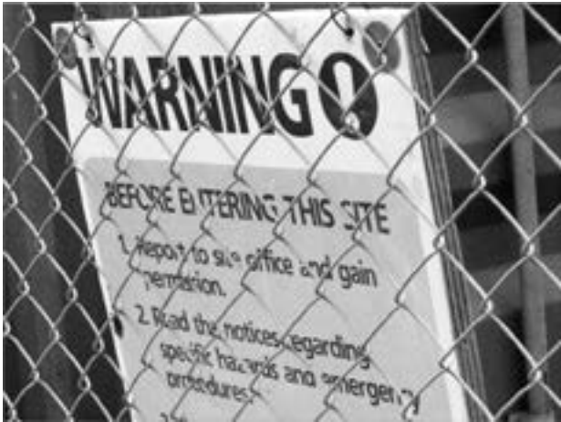
Good fencing and warning notices protect the public from hazards on this site.
