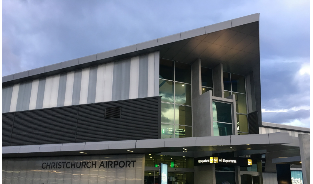
Christchurch International Airport. 4,500 m 2 of 1.5 mm Grey Butynol used for flat roof areas and gutters. Completed in 2013.
