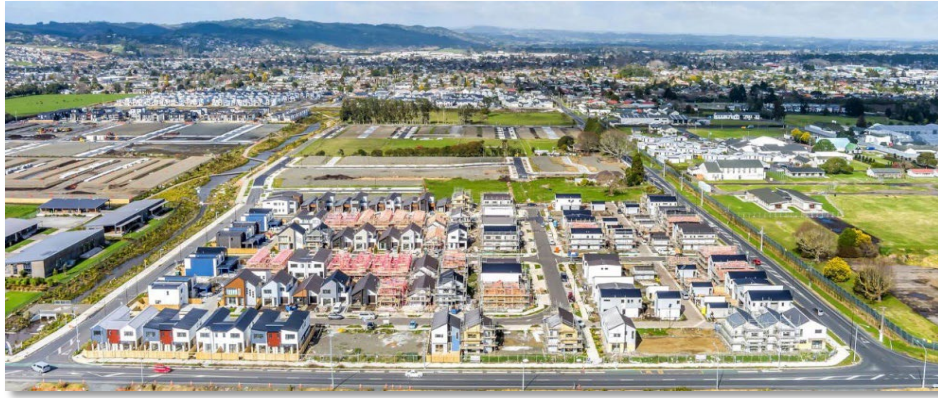
Figure 4.10 The construction site for the trial – reproduced with permission of the photograph owner
