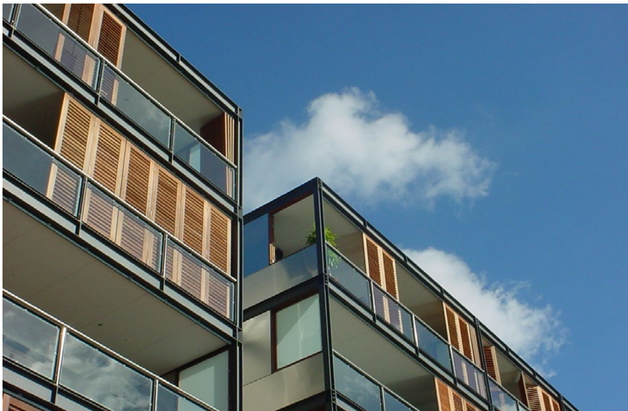
Glass barriers must be safety glass that meets the requirements in section 22 of NZS 4223.3:2016 and B1/AS1.
