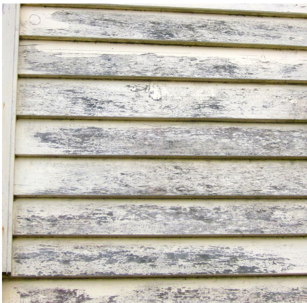
Examples of paint failure.
