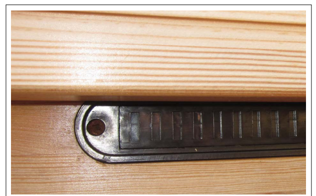
Trickle ventilator set in a window.
