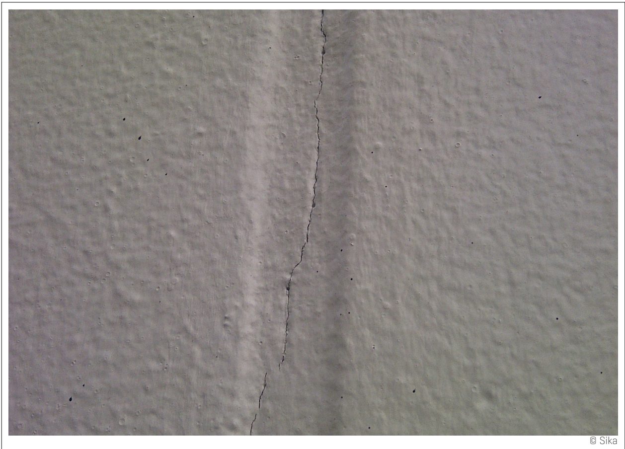
Cohesive sealant failure - sealant fracture.
