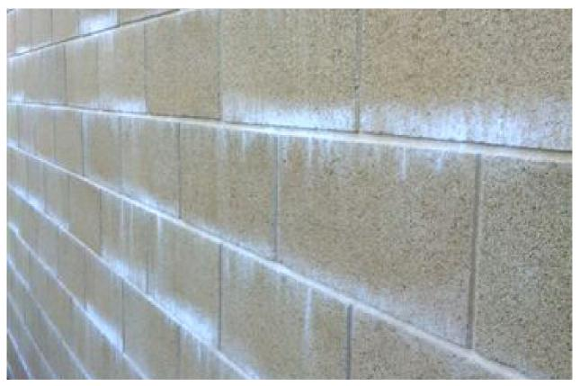
Figure 2. Salt deposits resulting from water in the wall exiting above each horizontal mortar joint.
