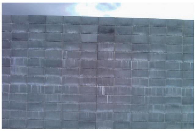
Figure 1. Typical efflorescence pattern on exterior concrete wall.
