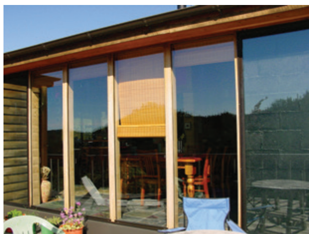
Trombe walls (left- and right-hand sides) and solar gain glazing in Ball House, Takaka (photo courtesy of Mark Fielding, Ecotect).
