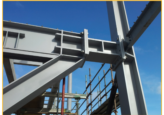
Eccentrically braced frame. (Source: Ruamoko Solutions.)
