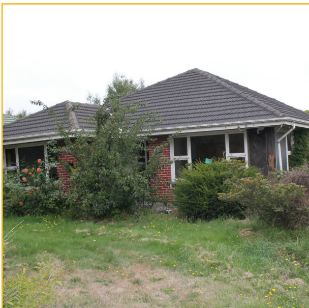
Settlement of the ground due to the compaction of the underground soil.
