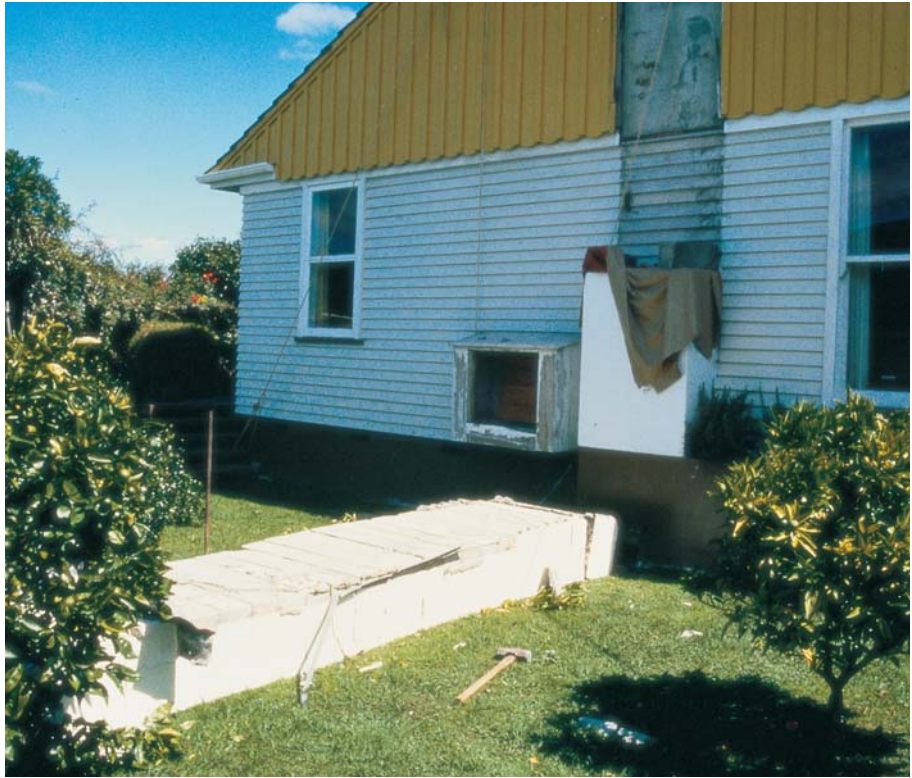
Figure 22: Many precast concrete chimneys collapsed. External chimneys that were not well connected to the buildings generally fell outwards. The Acceptable Solution B1/AS3 to the Building Code requires masonry chimneys to be reinforced and tied to the building at roof level. NZS 3604 provides for the extra bracing demand on the building structure. The introduction of these requirements mean that there should be much less failure than evidenced in the Edgecumbe earthquake.
