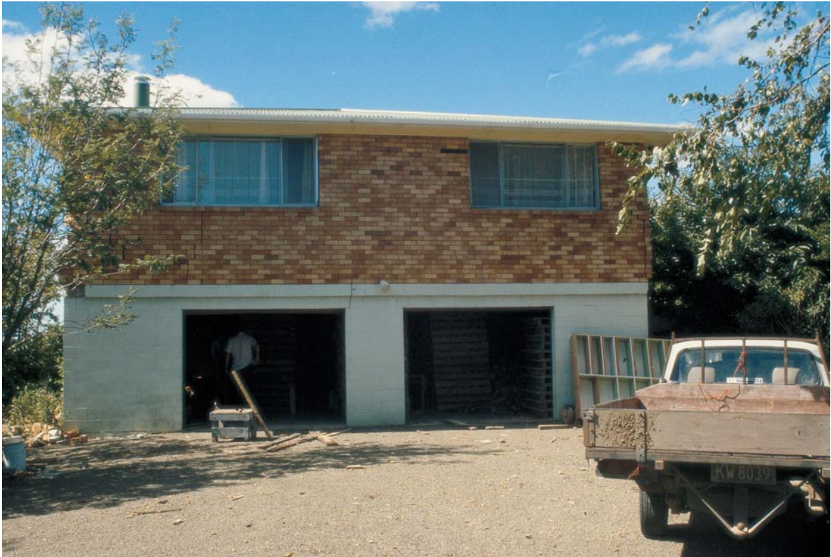
Figure 15: Reinforced concrete masonry structures generally performed well. Among those that did not, was this house built in the mid 1960s on the Rangitaiki Plains. Some cracking of the concrete masonry lintel beam and the brick veneer can be seen on this elevation.
