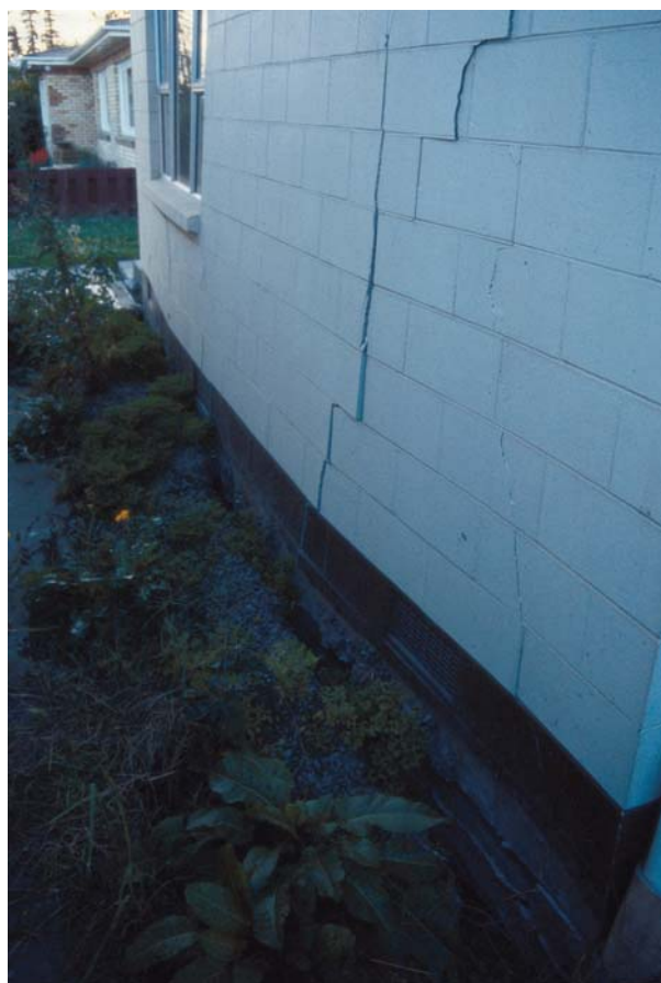
Figure 9: The damage to this wall of a block of three flats occurred when the flats moved as a unit and compressed the soft ground adjacent to the end of the walls. When the building stopped moving, the corners of the end wall (which were connected to the sidewalls) had returned to their original position, but the centre of the end wall (which was not connected to the floor) remained displaced.
