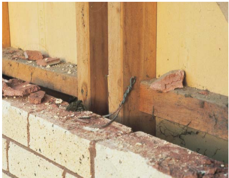
Figure 17: This type of wire tie, which was in common usage, is no longer permitted. As can be seen, they did not succeed in their role of tying the brick veneer to the timber-framed wall.
