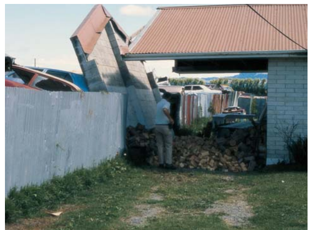
Figure 21: This masonry firewall on a boundary did not have adequate fixing to the roof framing or a foundation from which it could cantilever and stand alone.
