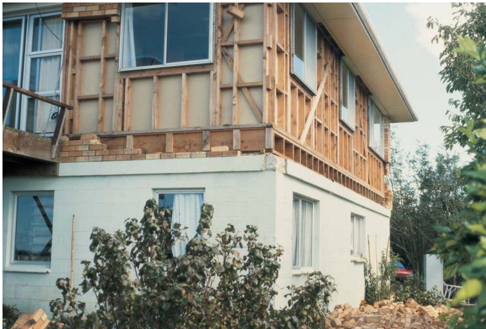
Figure 18: A view of the rear of the house reveals the extent of the brick veneer failure. Note that the windows have remained intact despite the severe shaking the building has suffered.
