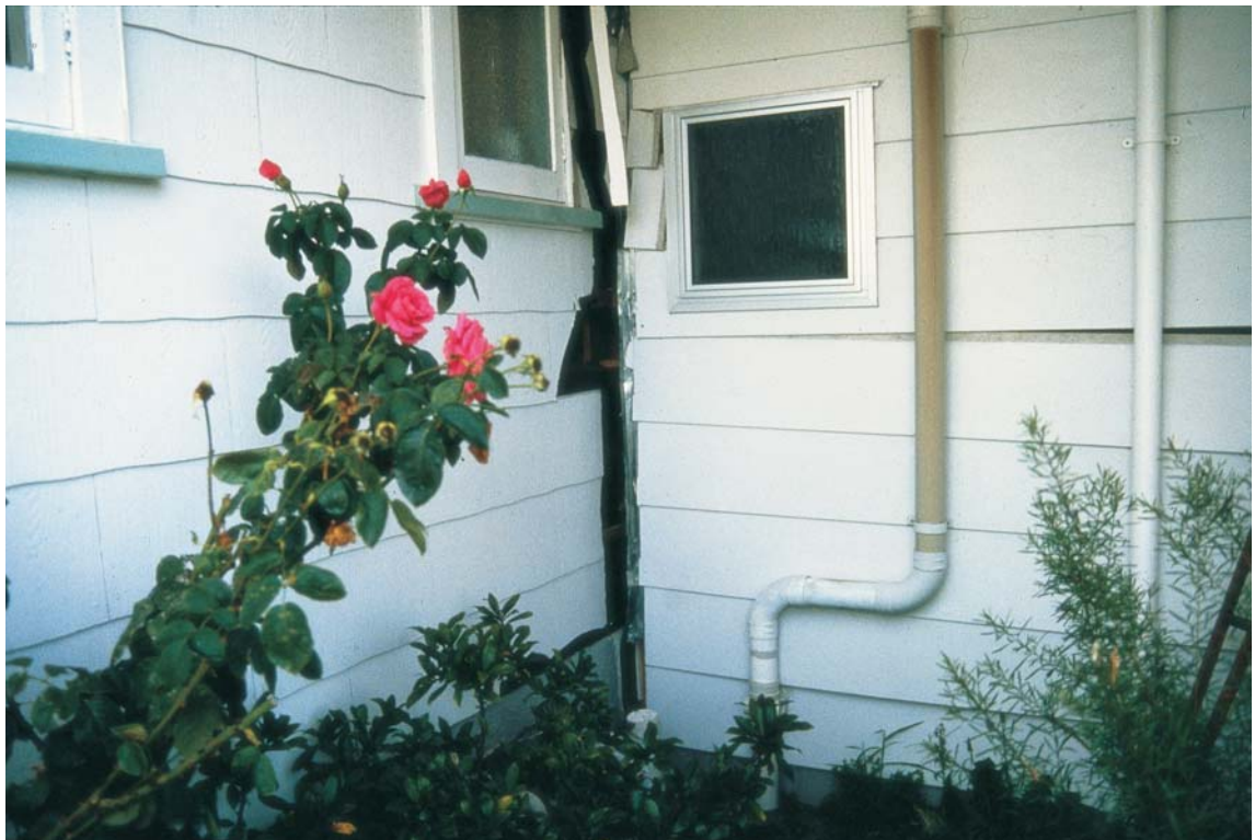
Figure 11: Some houses and additions were built partly on piles and partly on slab-on-ground. Often there was damage at the junction between these types of construction because each type moved differently. This is a particularly vulnerable feature of alterations and additions if there is not adequate connection between the old and the new.
