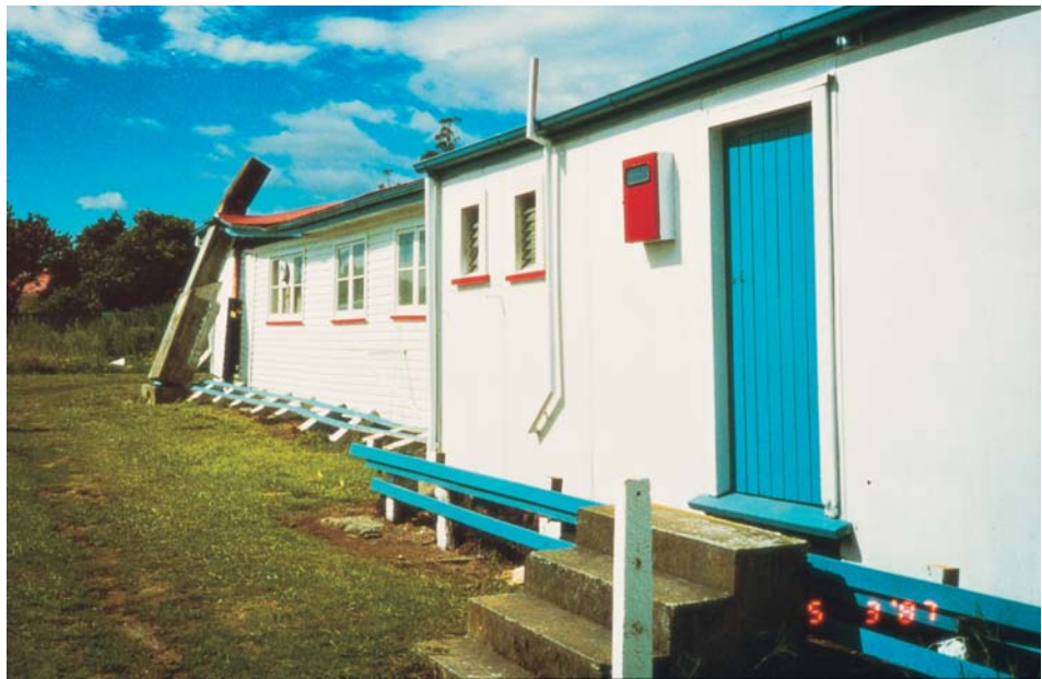
Figure 4: Ordinary piles are not able to resist lateral loading. Anchor piles or braced piles are now required for this purpose. The Te Teko Returned Services Association Hall rolled over on its piles, while the chimney base and steps remained in place.
