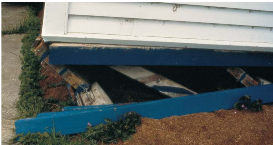
Figure 3: This subfloor consists of concrete piles with jackstuds. This detail would not comply with the bracing requirements of NZS 3604. The number of braces and the nature of their connections in this house were insufficient to withstand the imposed earthquake load from the house. (This is a close-up of the house shown in Figure 2)
