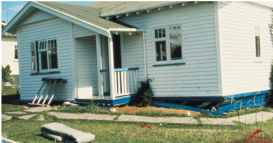
Figure 2: Many anomalies were seen and probably resulted from the effects of variable soil conditions giving rise to differing building movement in the earthquake. A near identical house next door to this one remained on its foundations and largely undamaged.
