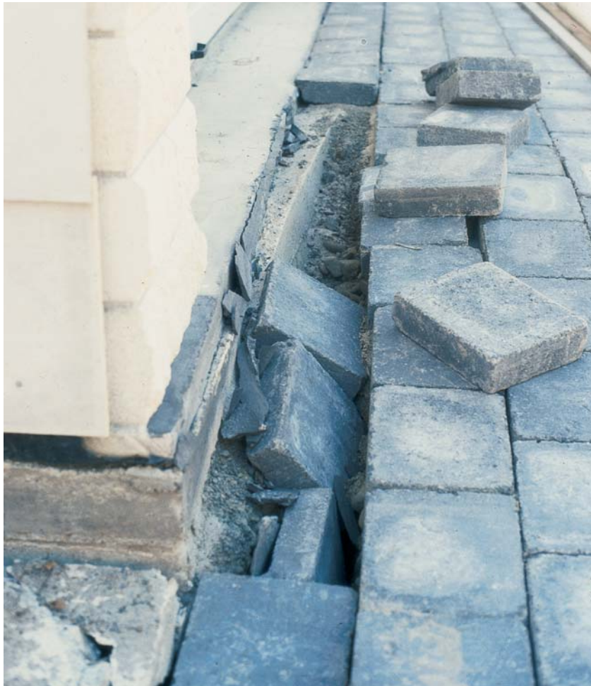
Figure 12: Soft ground in the area resulted in subterranean movement. The floor slab of this garage moved laterally, displacing the adjacent paving slabs.
