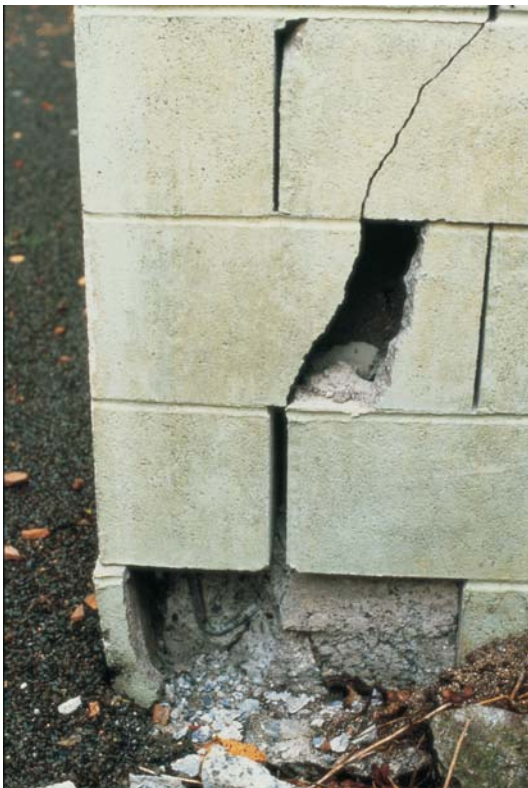
Figure 16: The lower storey concrete block masonry was reinforced both horizontally and vertically with plain mild steel rods. Despite the reinforcing, cracking occurred in several places at the corners.
