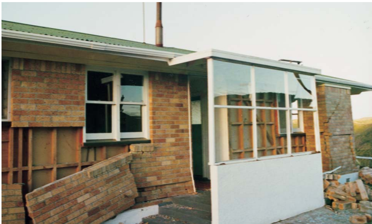
Figure 7: This house, on the foothills at Awakeri, suffered substantial damage to its foundations and brick veneer. The floor system was independently supported on unbraced piles and was not tied to the perimeter walls. Lateral displacement of the house battered the veneer, dislodging it from its seating on the perimeter wall.
