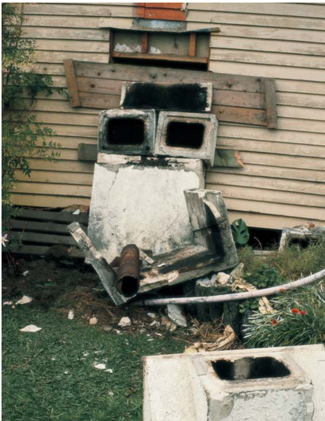
Figure 23: Many chimneys that failed were found to have no reinforcing in them, and the individual elements separated as the chimney collapsed.
