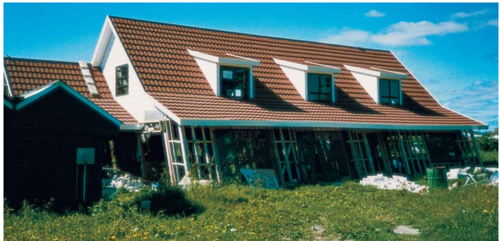
Figure 26: Unlined houses are particularly vulnerable to lateral loading from either earthquake or wind actions. The contribution of the internal linings to the resistance to lateral load, and the need to ensure adequate nailing of the lining, is shown by the near collapse of this unlined house.
