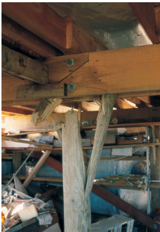
Figure 29: The pole supports acted as cantilevers and were unbraced. This internal pole, fractured below the beam. The split-level floor reduced the effectiveness of the floor diaphragm action. NZS 3604 now requires a bracing line at all discontinuities of the floor level.
