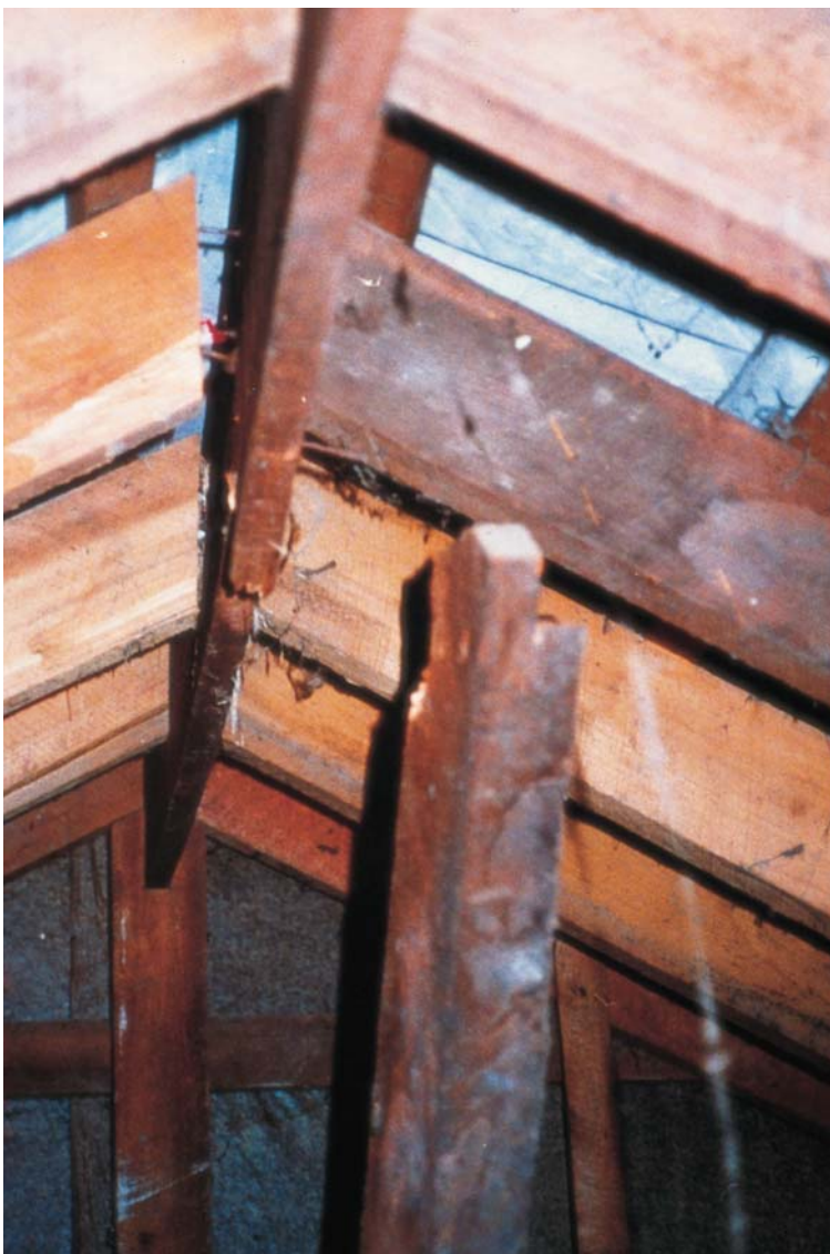
Figure 32: In this gable-ended concrete tiled roof, the nailed connections between the diagonal roof braces and the ridge board failed. The end of the brace was fixed to the ridge board directly below a rafter. When the brace was loaded in compression, it raised the ridge board, pushing the rafter out of place.
