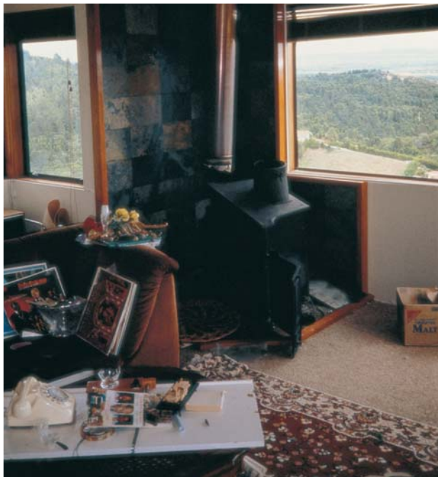
Figure 25: Wood-burning stoves, both free standing and in-built, were displaced by the earthquake. The need to adequately fix these appliances to the floor was clearly demonstrated as many stoves were standing on smooth hearths and when shaken they moved easily, tearing free from their flue and, in some instances, tipping over and spilling the contents of their fire boxes.
