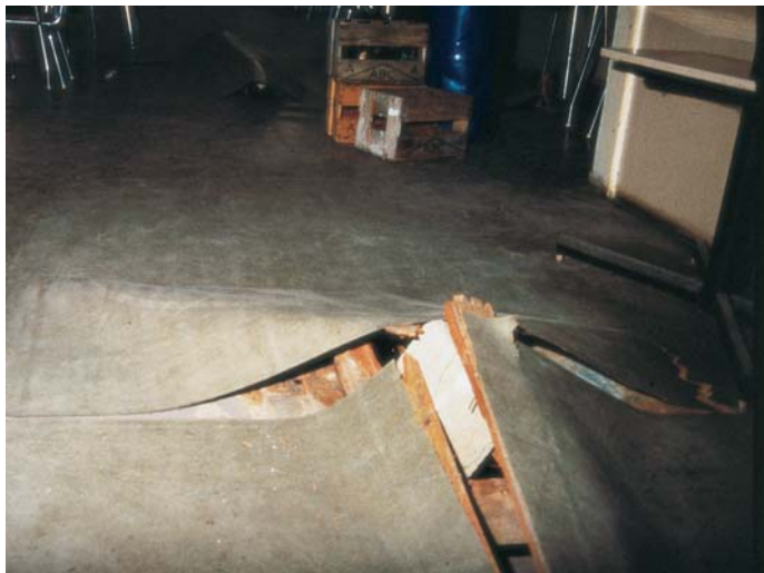
Figure 5: The floors of several structures which fell off their foundations, were punctured by interior piles that remained upright as the building fell.
