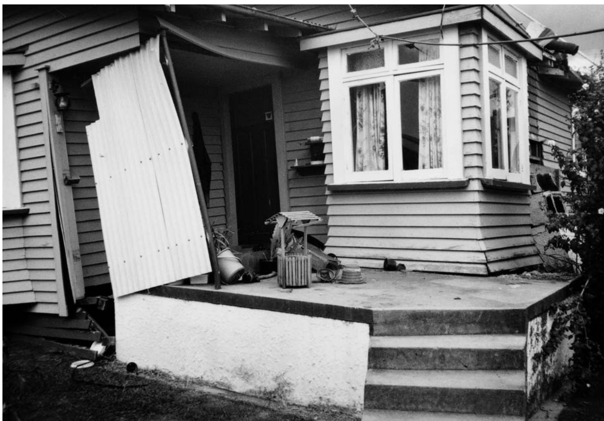
Figure 1: Houses built before NZS 3604 frequently used unbraced piles and jackstuds. Movement and partial collapse was common with about 30 houses moving on their foundations. The result was that many seriously damaged their superstructure and services.
