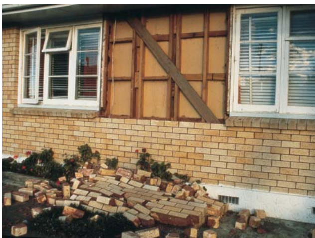
Figure 20: Brick veneer panels between windows were particularly vulnerable, yet the windows nearly always remained intact.
