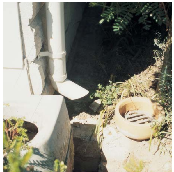
Figure 14: Ground movement often caused surface cracking. A slab-on-ground 'L' shaped dwelling was crossed by a significant fissure and the slab has split by about 100 mm. Minor settlement also occurred around the property, resulting in reverse fall of gutters, etc. It is not practical to build domestic buildings to resist this sort of damage.
