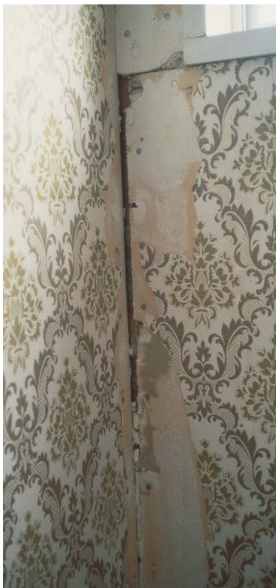
Figure 30: Walls of different height moved differently, often resulting in cracked wall linings and fractured plaster joints.
