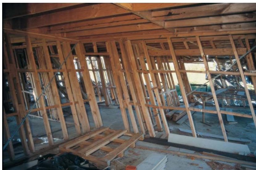
Figure 27: Inside the house the internal metal angle braces were insufficient to handle the earthquake loads from the relatively heavy upper-storey.
