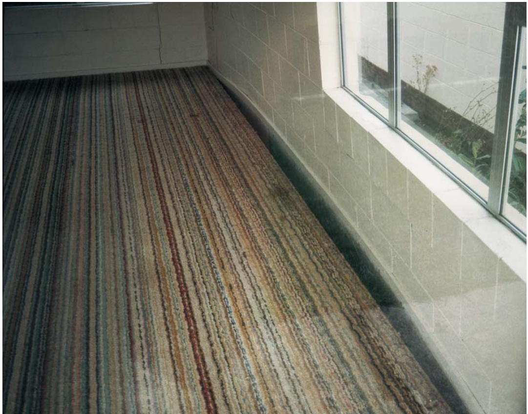
Figure 10: NZS 3604 and NZS 4229 still permit floor slabs not to be connected to foundation walls for single-storey buildings providing they are 'contained' within the foundation walls. Here, the floor in the flats (refer to Figure 9) has separated from the end wall when the middle of the wall has not returned to its original position, leaving a significant gap.
