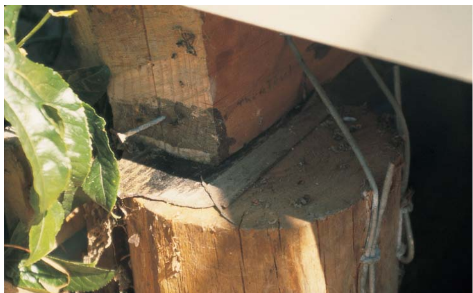
Figure 6: Some houses were founded on driven timber piles to overcome soft foundation conditions. Movement of up to 50mm was observed between the bearers and the piles. NZS 3604 requires a 6kN connection in this situation, which clearly was not provided here. This connection is one that is still commonly not carried out correctly, even in houses built today.
