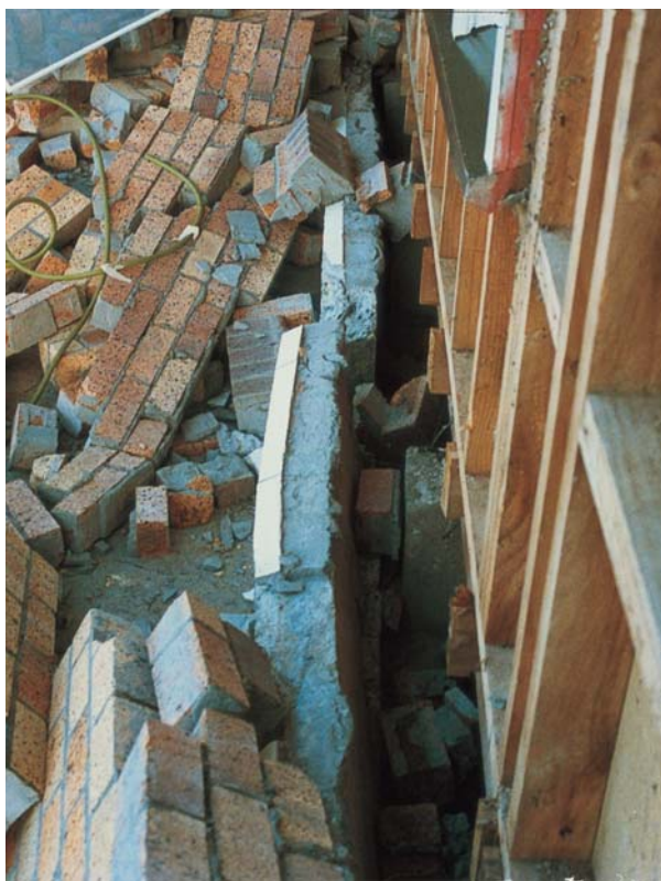
Figure 8: Provisions for lateral support of foundation walls are intended to prevent this happening. The joists should be connected to a plate bolted to the top of the foundation wall.
