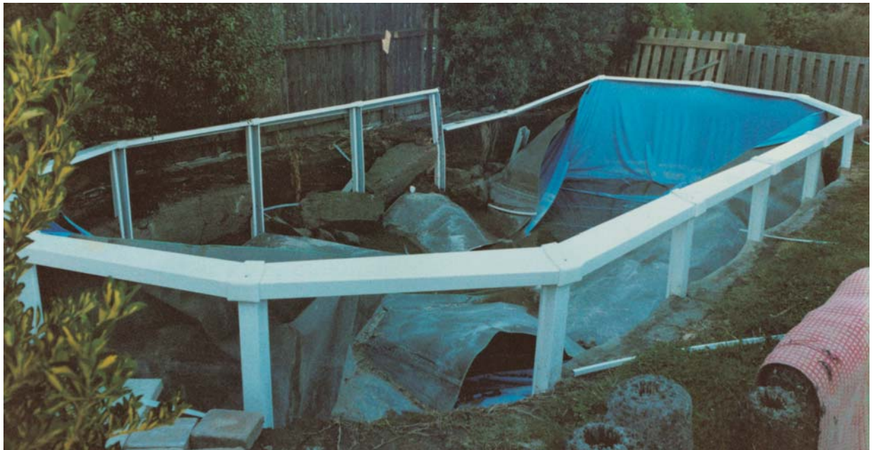
Figure 31: Water-containing structures experienced substantial damage during the earthquake. Many pools were badly damaged in the area. Water was described as being 'thrown' from pools in Edgecumbe.
