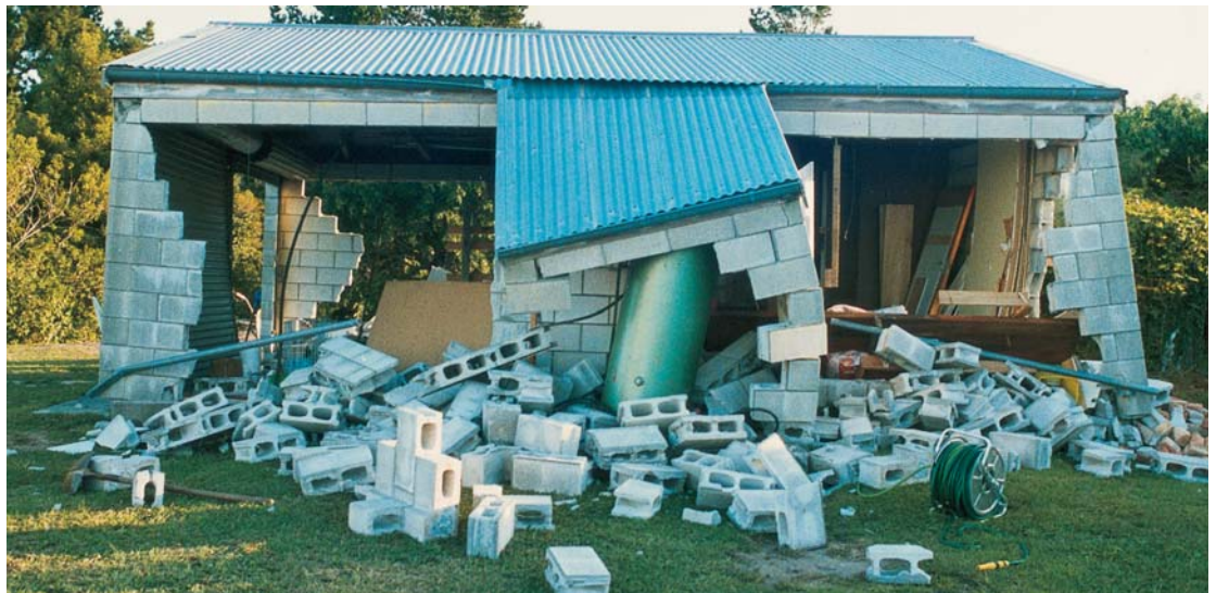
Figure 19: The minimum reinforcing requirements of NZS 4229 are intended to prevent the total disintegration of masonry structure as shown here.
