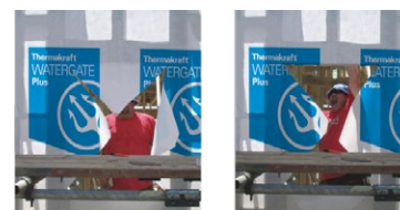
On arrival of doors and windows, cut Watergate at each opening on a 45° angle away from each corner. Pull the Watergate flaps inside and fasten to the inside of frame.
