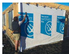
Fix Watergate Plus securely to the frame.
