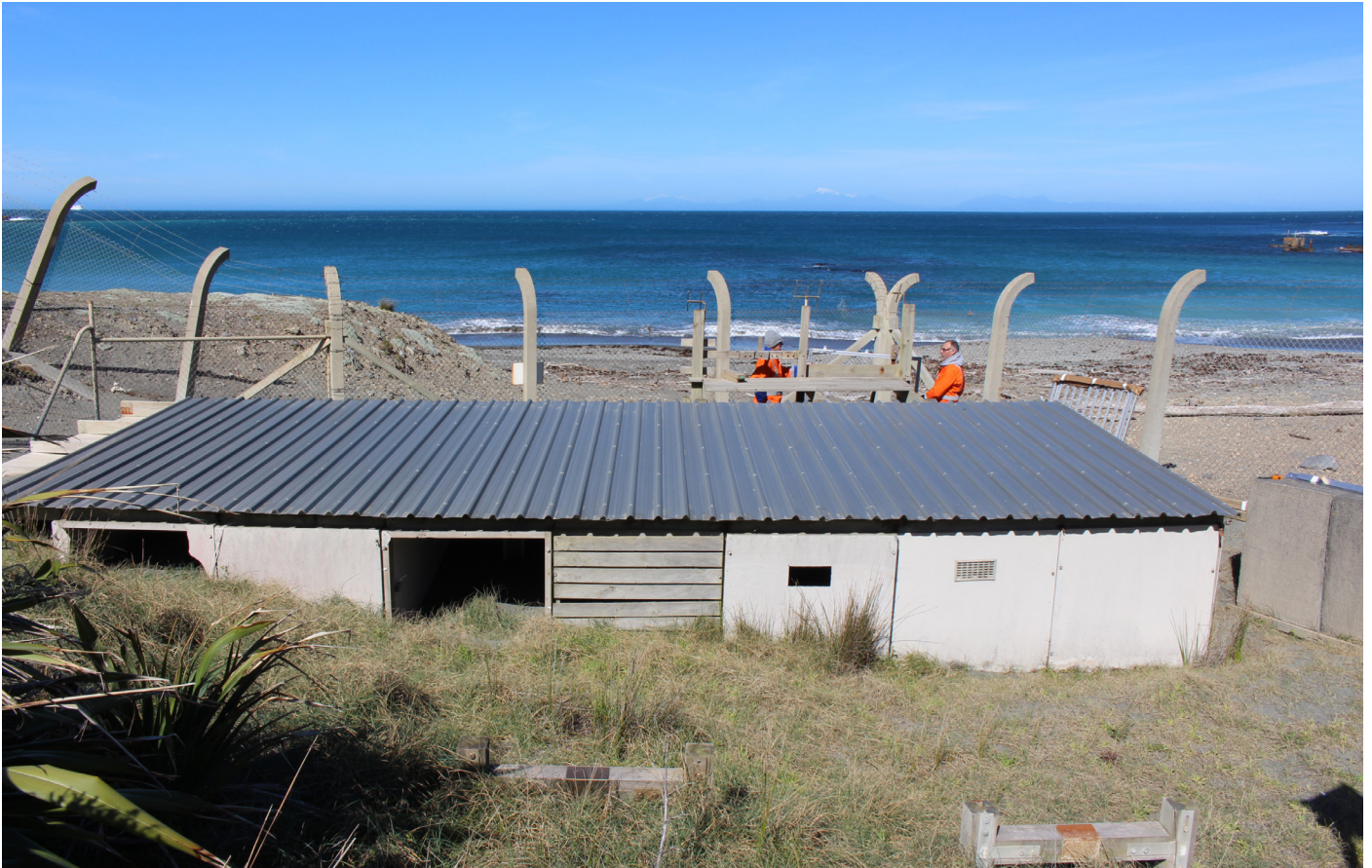
Figure 1. Test structure located on the south coast of Wellington used to measure rates of corrosion of steel samples placed in the roof cavity.
