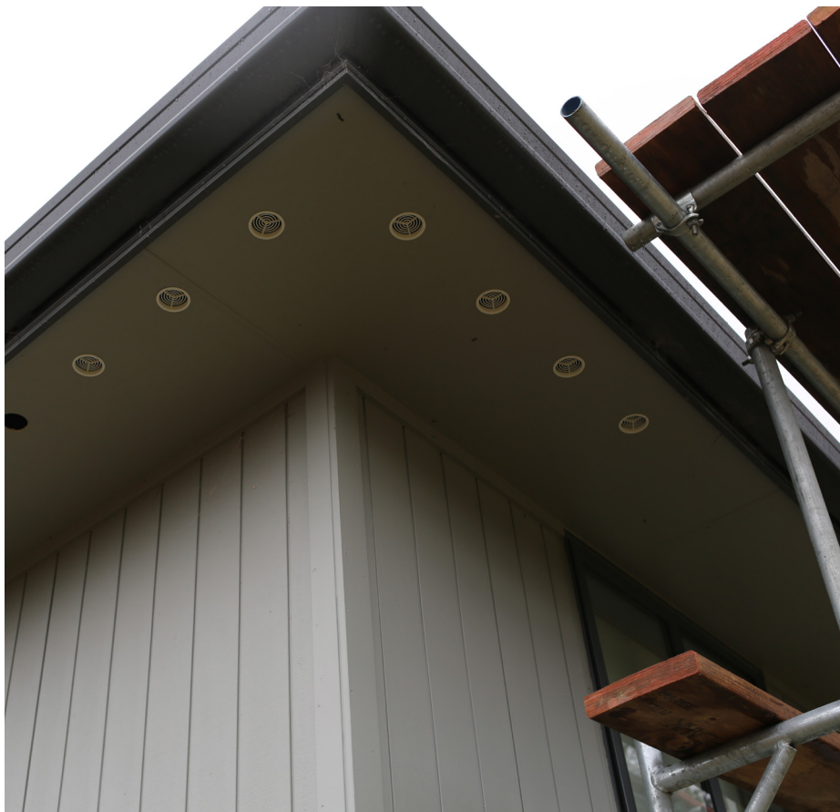
Figure 2. Example of circular soffit board vents during construction.
