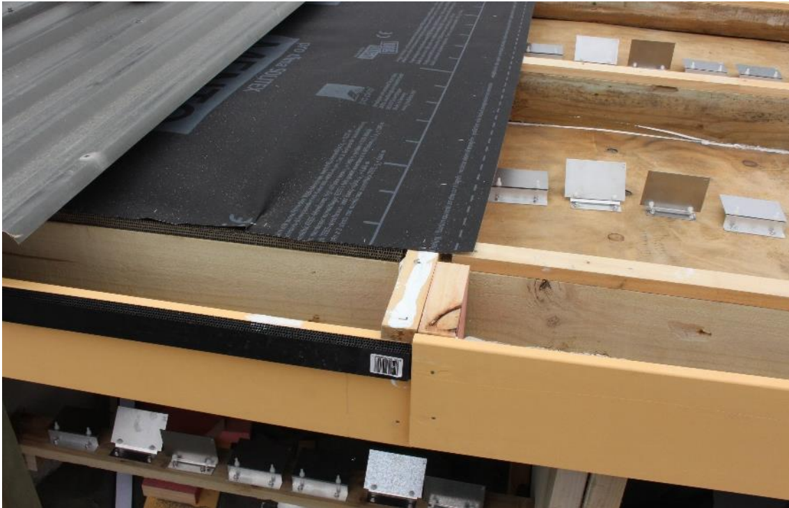
Figure 5. Roofing underlay being installed over the vented cavity.
