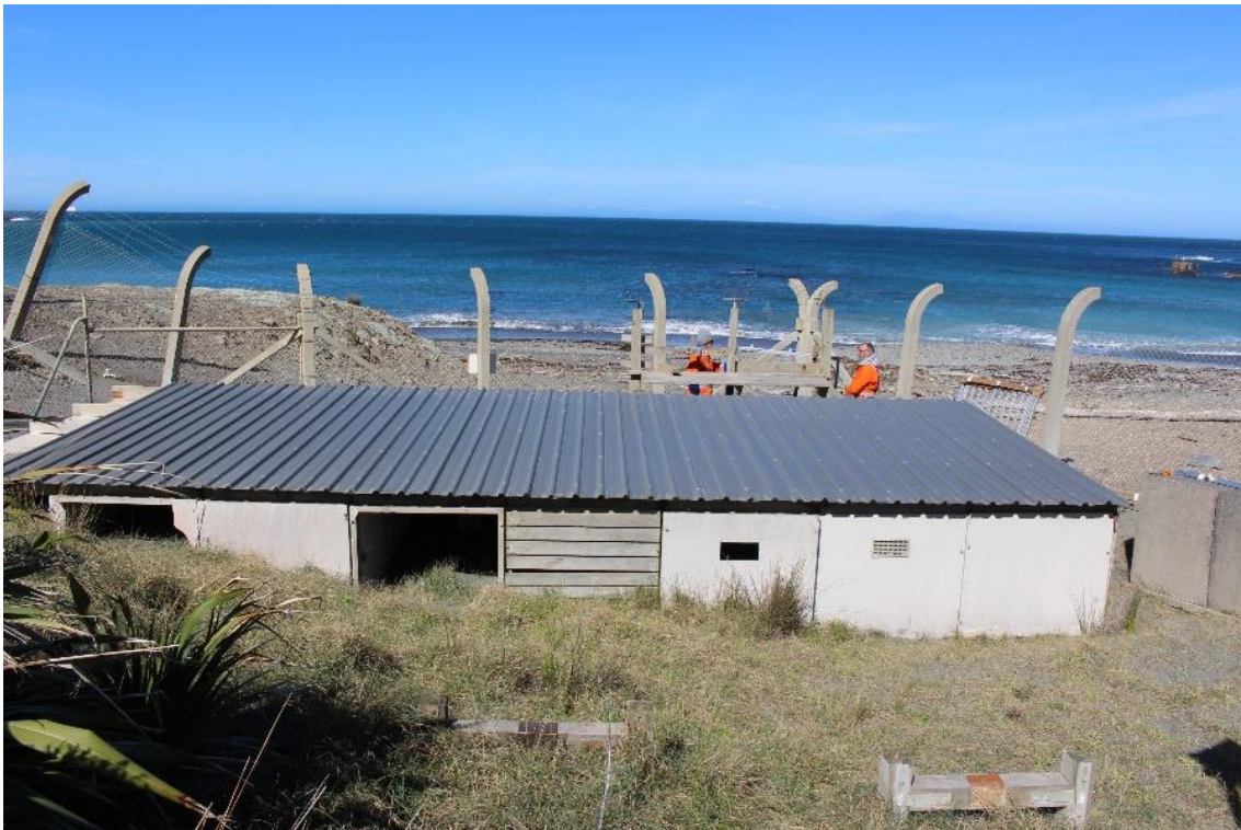
Figure 1. Test structure located at the remote south coast of Wellington.
