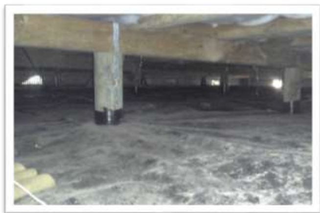
Figure 22. A ground cover is important for preventing ground-sourced moisture entering the home.
