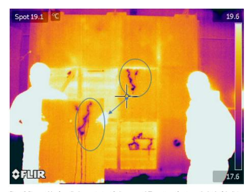
Figure 2. Disassembly of a wall where water transfer has occurred. The pattern of water on the back of the lining being held up matches the pattern on the surface of the insulation.
