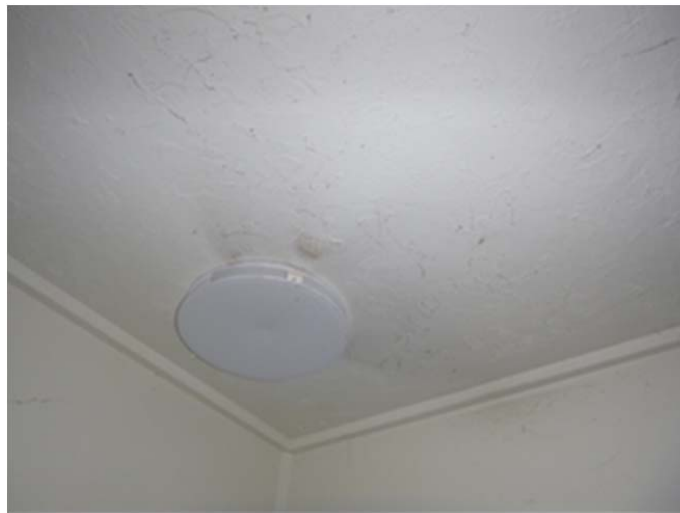
Figure 46: Discoloration around the outlets of a DVS system indicating a need for maintenance
