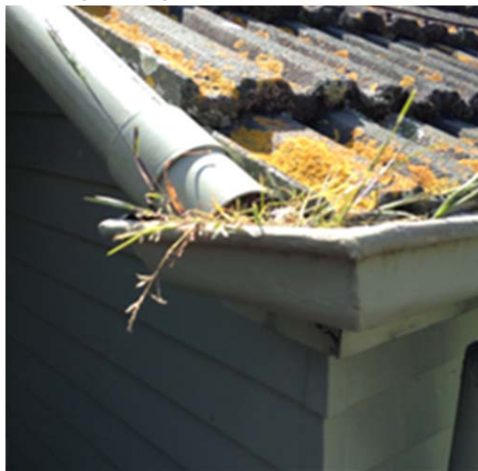
Figure 39: This blocked gutter was causing water to rot the bargeboard (underneath gutter) and allowing water to enter the wall cavity
