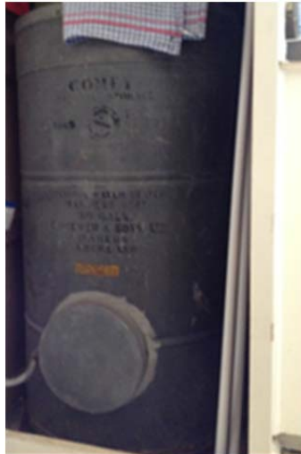
Figure 26: Some cylinders were very old and required replacement in the near future - note also the lack of cylinder wrap and pipe lagging
