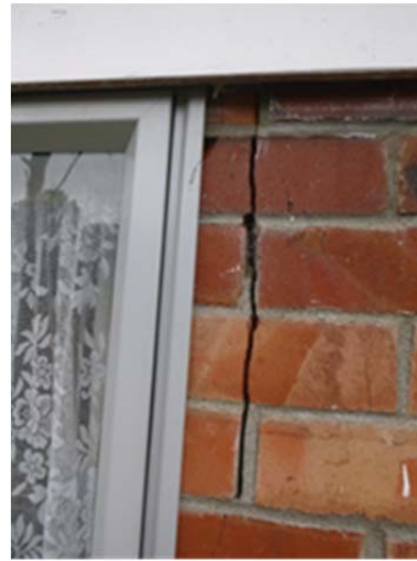
Figure 12: Damage to brickwork from DIY installation of a window
