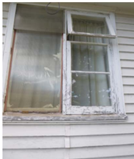
Figure 15: A window requiring significant repair following a lack of maintenance (primarily painting and avoiding rot)
