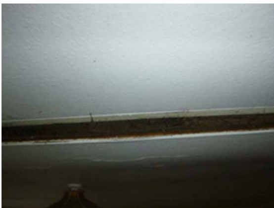
Figure 35: Bow in the ceiling caused by the damp pinex
