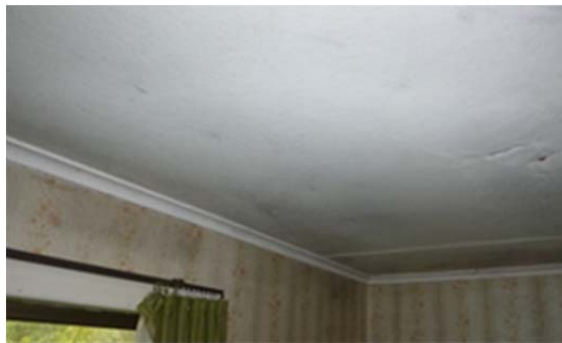
Figure 34: Damp pinex ceiling caused by a roof leak
