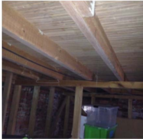
Figure 20: A simple underfloor insulation job waiting to happen. Good access with the potential to achieve a good result.
