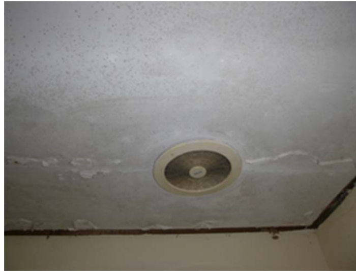
Figure 29: A less than adequate bathroom extract leading to mould and deterioration of the painted surfaces on the ceiling and wall
