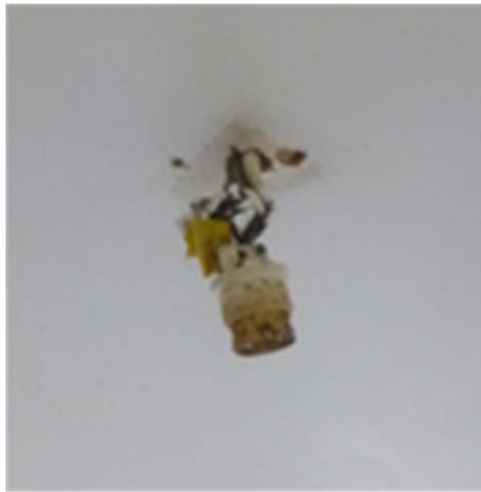
Figure 42: This light fitting is dangling precariously from the ceiling and is potentially unsafe
