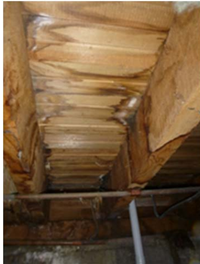
Figure 23: The underside of a floor indicating significant damp rising into the structure of the house from the sub-floor area
