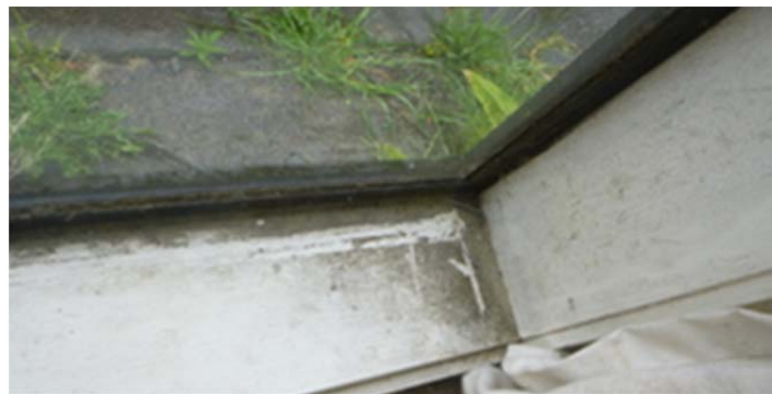
Figure 17: An aluminium window with perished rubber seals allowing moisture ingress - note the mould
