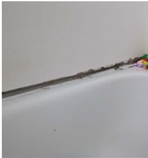
Figure 37: The seal has been removed from this bath and the silicone has deteriorated causing additional and unnecessary moisture issues in the home
