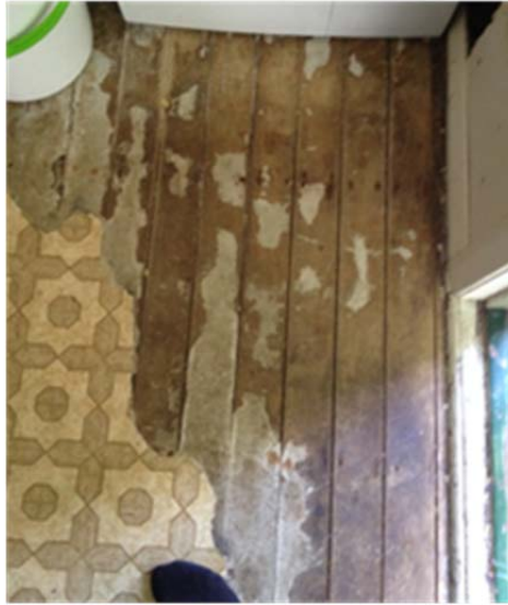
Figure 33: Lino on a kitchen floor which needs replacing
