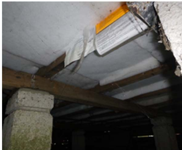
Figure 21: An underfloor that has benefited from EECA's Warm Up NZ installation of bulk underfloor insulation - note the labelling and information provided
