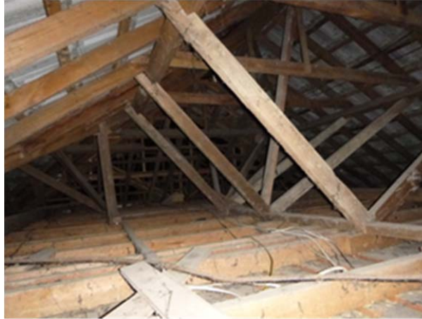
Figure 44: Wiring in this house is a combination of old style perishable wiring that may be a safety risk and new wiring
