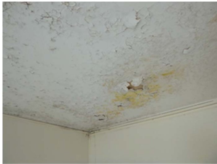
Figure 32: Significant deterioration of internal paintwork leading to the start of breakdown in the plasterboard
