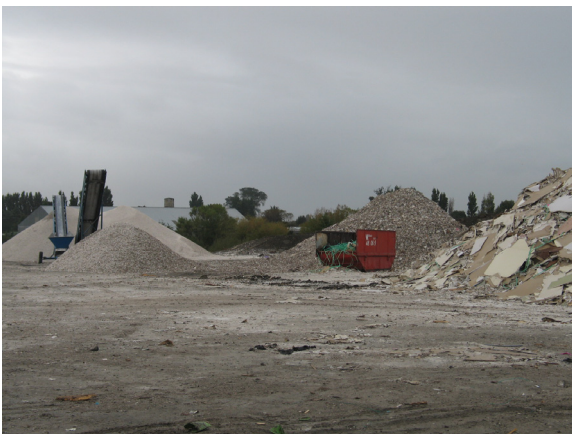
Stockpiles of crushed gypsum and paper and, contamination skip at Crusaders Landscaping, Christchurch.
